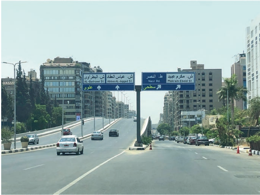
Fig. 7 A newly erected flyover in Nasr City. Source: Author. Date: 11 July 2021
