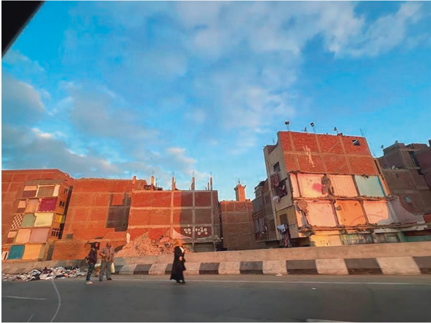
Fig. 5 Ring Road demolitions. Source: Author. Date: 19 February 2023
