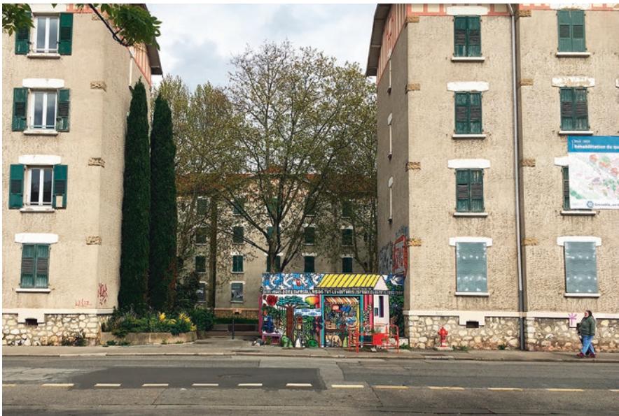
Fig. 3 Temporary housing in the Abbaye urban renovation scheme, Grenoble. Source: Author, 23 April 2023
