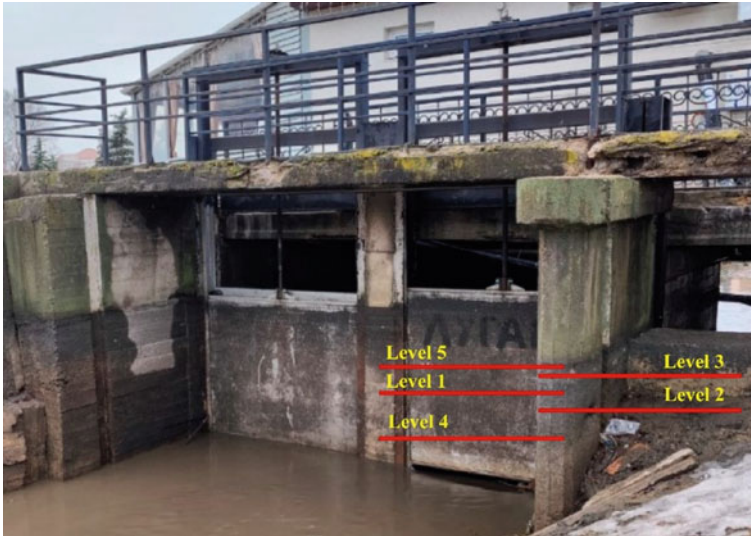
Fig. 20.5 Water stages of Komsomolsky pond while the automatic level maintenance system operates. Lv. 1 represents the highest calculated water level in the pond (turning off the pump), Lv. 2 represents the lower calculated water level in the pond (turning on the pump), Lv. 3 illustrates the level at which the shield gate opens, Lv. 4 represents the water level with an unfavorable precipitation forecast, and Lv. 5 represents the stable water level with the mean annual discharge
