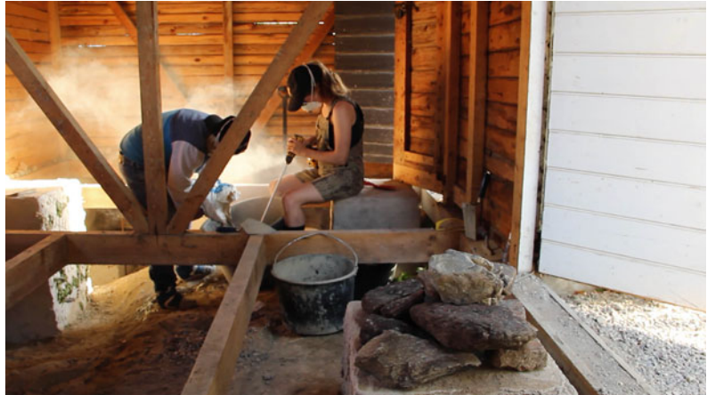
Fig. 3.3 Mixing mortar
