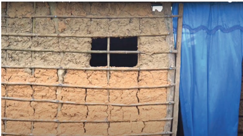
Fig. 2.4 Photograph from the documentary. La Victoria neighborhood, El Nispero, Montes de María, 2021. Window in a “bahareque” house, the Afro-Caribbean
