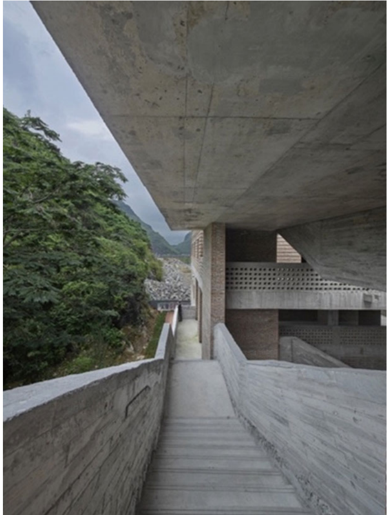
Fig. 8.11 Staircase from exterior
