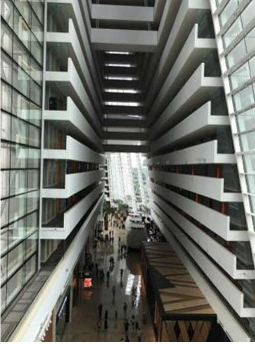
Fig. 1.1 Ground floor and atrium of Marina Bay Sands Hotel. Source author
