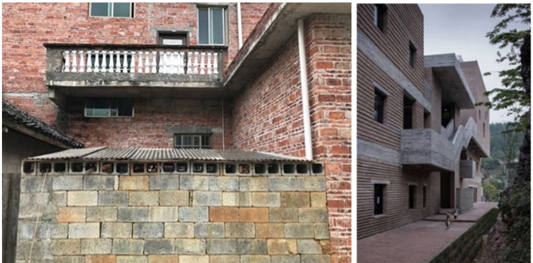
Fig. 8.19 Local red bricks and hollow concrete blocks, we also continue this combination of materials in the new building
