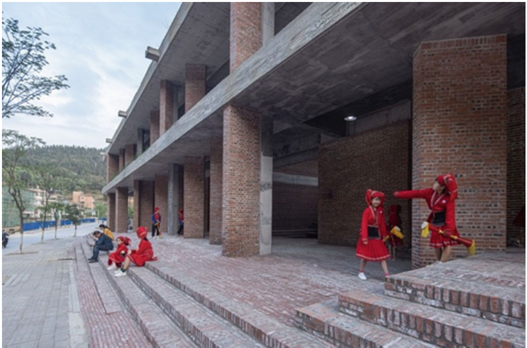
Fig. 8.6 Gables and steps
