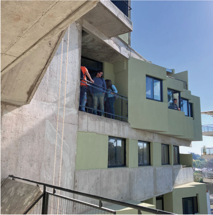
Fig. 26.27 Under construction: visit of university students to the Biarritz building
