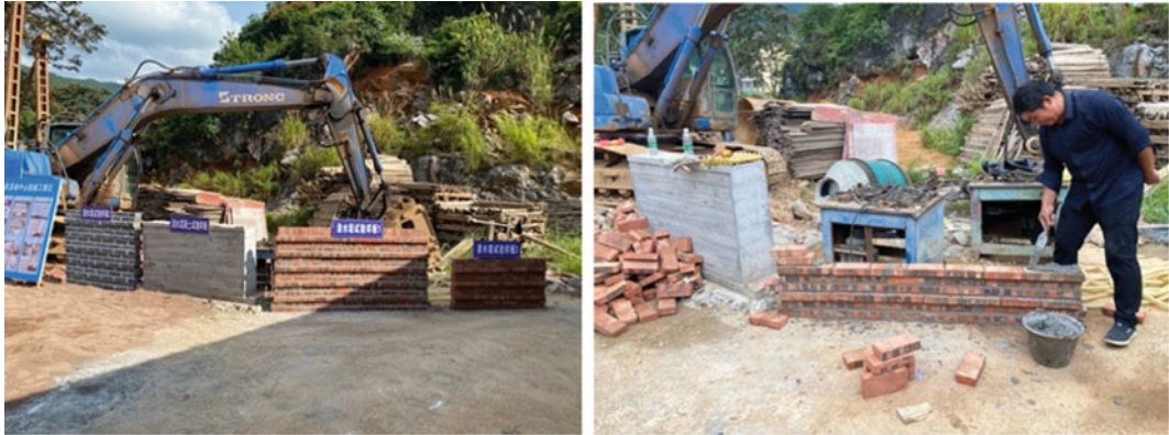
Fig. 8.20 Local red bricks and hollow concrete blocks
