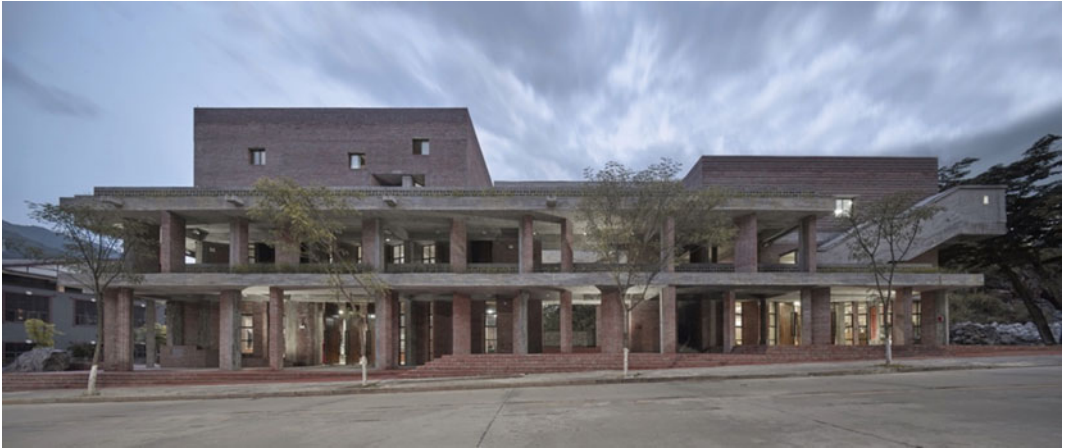
Fig. 8.7 Main entrance facade real view
