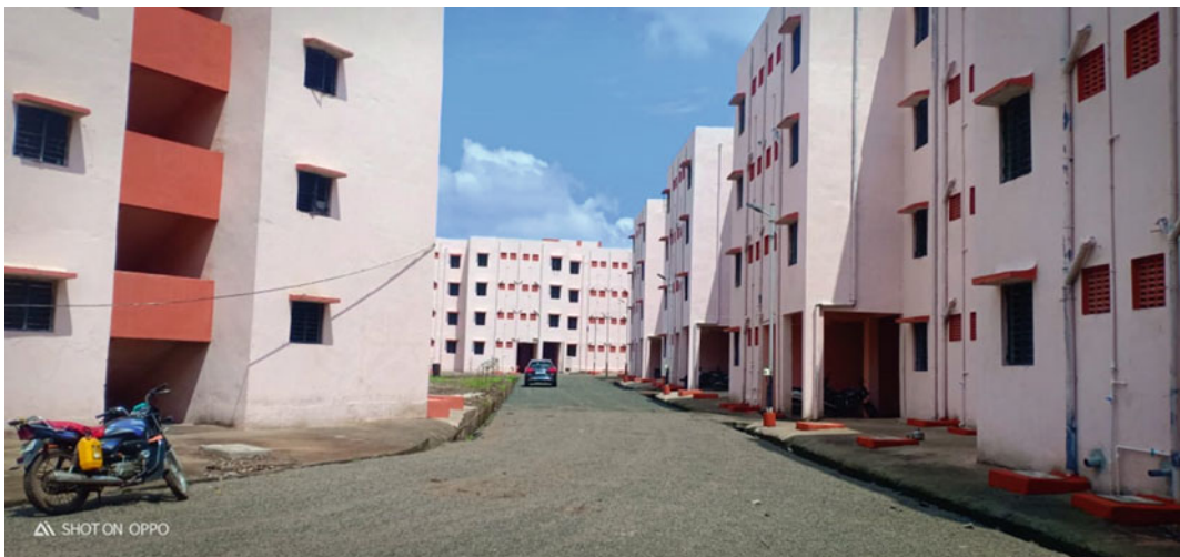
Fig. 5.4 IHSDP Housing project—view of the society
