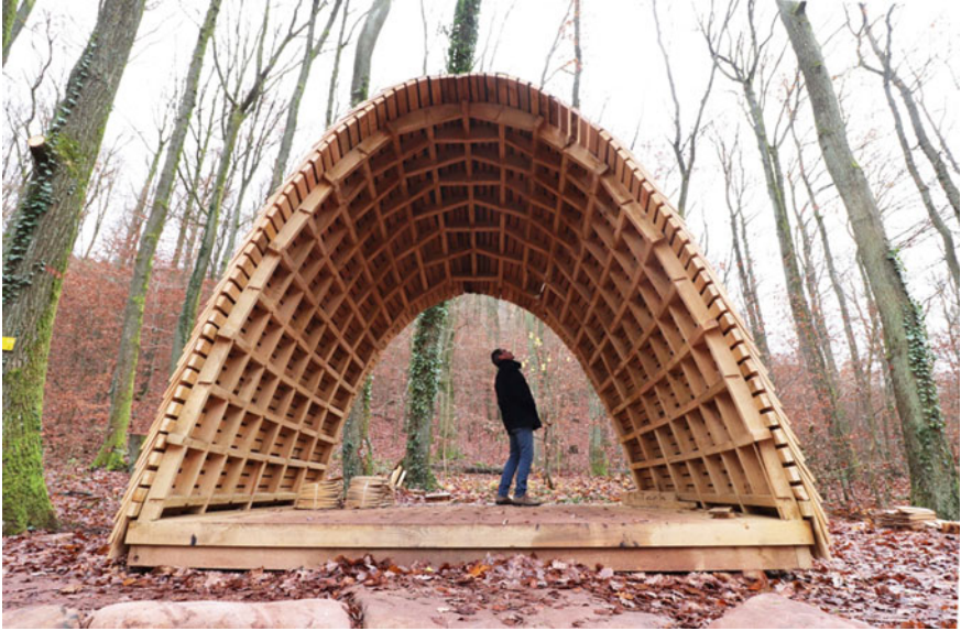
Fig. 9 Completed structure with sweet chestnut flooring and roof cover
