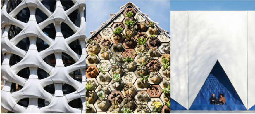
Fig. 2 Additive manufacturing: Arachne 3D printed facade (©Archi-Solution Workshop); House of 3D Printed Curiosities (©Matthew Millman Photography/Emerging Objects); EU Building 3D printed facade (©Ossip van Duivenbode)
