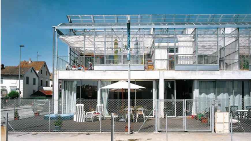
Fig. 15 Exterior view of Lacaton and Vassal “Manifesto City”, in Mulhouse, France, 2014
