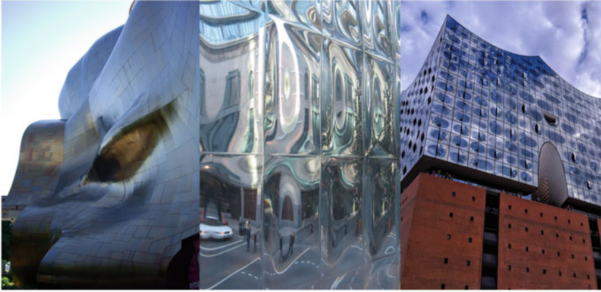
Fig. 4 Formative manufacturing: Experience Music Project (©Jon Stockton/CC BY-SA 3.0); Holt Renfrew flagship store in Vancouver (©Marc Simmons/FrontInc); Elbphilharmonie Hamburg (©Bahman Engheta/CC BY-SA 4.0)
