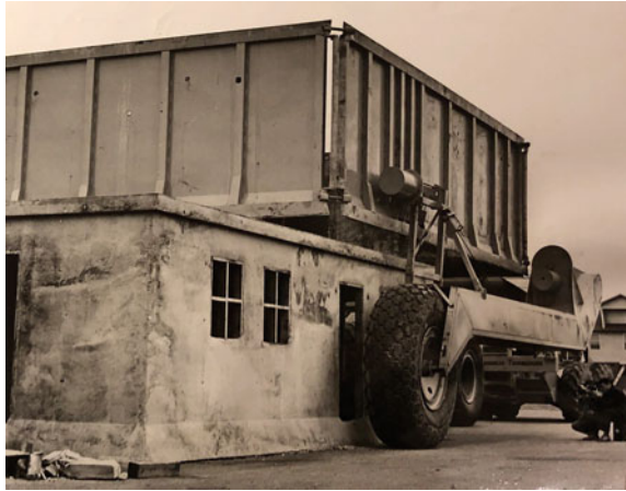
Fig. 4 Tournalayer—Outer Form for house form assembly (1955) R.G. Le Tourneau ( source Carlo Carbone private collection)
