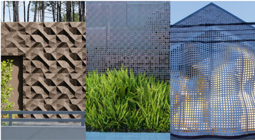
Fig. 3 Subtractive manufacturing: cork facade (©GenCork and Sofalca); De Young Museum (©David Basulto via flickr); MaoHaus facade (©XiaZhi)
