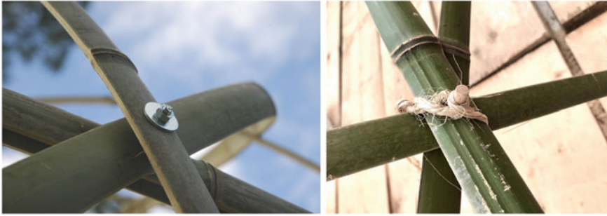
Fig. 7 Iron bolts (left) or timber pins with hemp rope (right) as node-connectors
