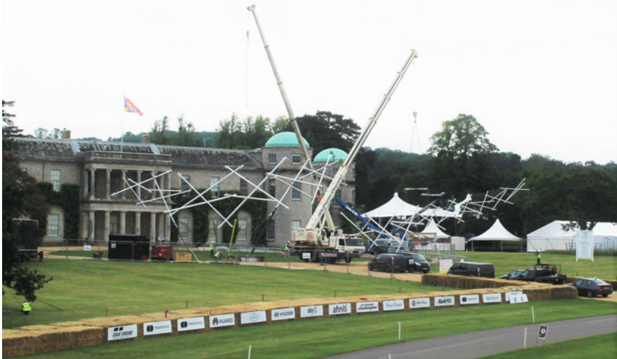
Fig. 8 The final part of the sculpture being lifted into place. Photo Credit The Goodwood Estate Company Limited
