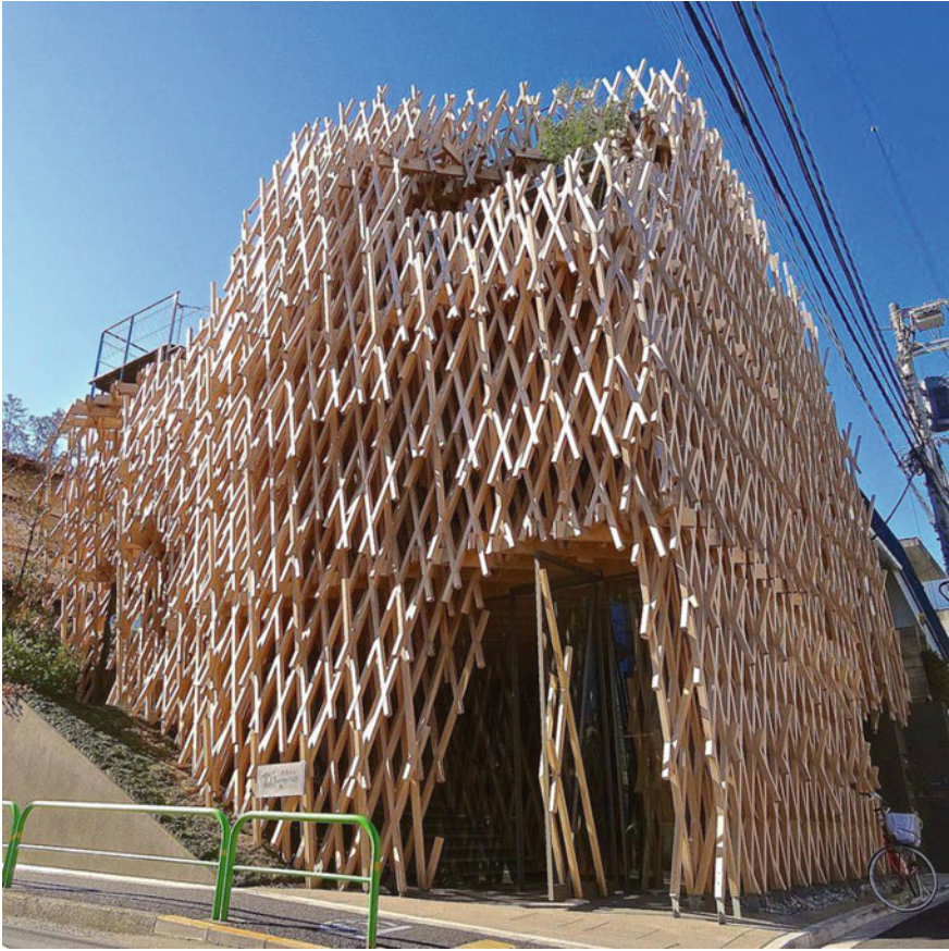
Fig. 5 Exterior view of Kengo Kuma's SunnyHills cake shop in Tokyo, Japan, 2013. Courtesy of Design Gallerist, Blog section https://www.designgallerist.com/blog/sunny-hills-kengo-kuma/
