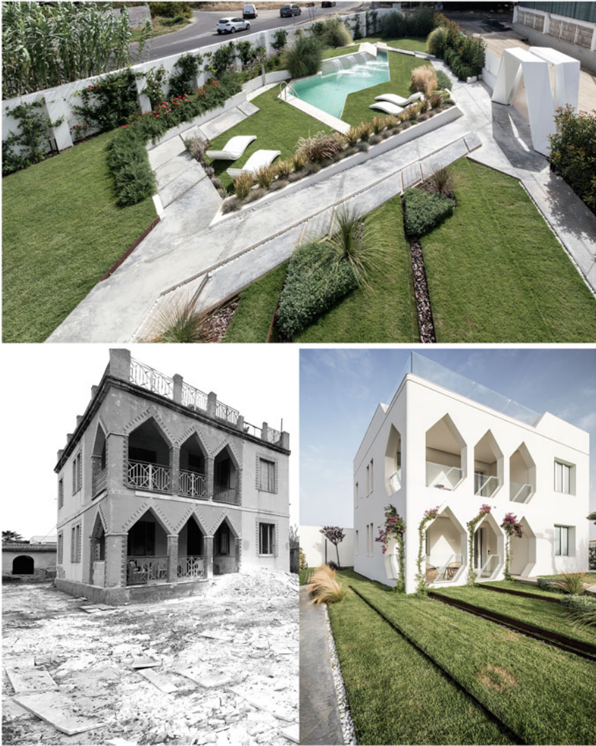
Fig. 1 a, b View of Villa Vi's main garden and building. A computational environmental analysis informed the differential organization of the landscape so to provide a beneficial microclimate for outdoor living during the hot summer season
