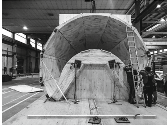
Fig. 7 Large-scale robotically fabricated timber formwork for free-formed concrete columns
