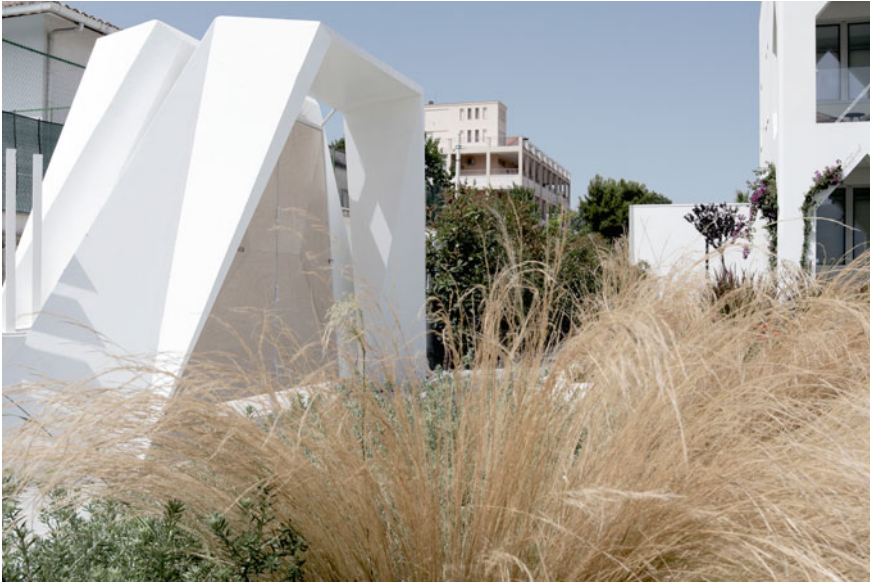
Fig. 5 Digital Concrete: a view of the FRC portal
