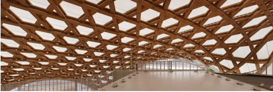
Fig. 3 Interior of the “wooden tent” designed by Shigeru Ban for Pompidou Metz Museum. The whole structure was controlled and fabricated through a lightweight digital model prepared by designtoproductio. v1—Photo by Didier Boy de la Tour, taken from AREA Magazine online. v2—Courtesy of Jean De Gastines Architects
