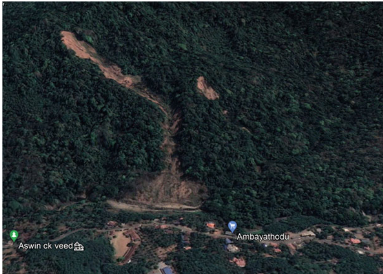
Fig. 17.6 Google earth image of landslide occurred at Ambayathode on August 16, 2017
