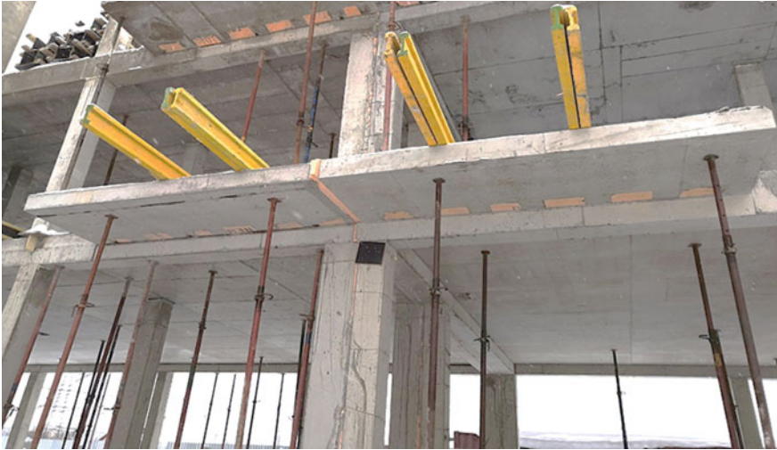
Fig. 1 Thermal pads in a monolithic overlap
