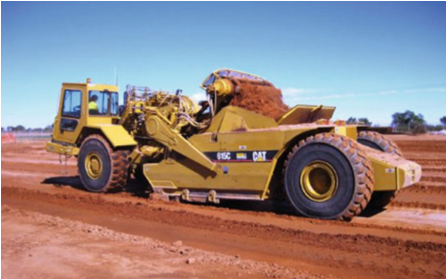
Fig. 1 Wheeled vehicles in construction
