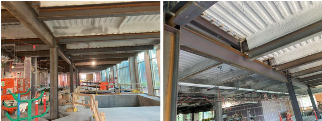
Fig. 33.7 Case 4 – Stiffening steel and new columns and girders
