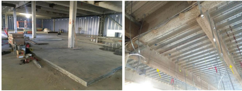
Fig. 33.5 Case 3 – Photos of topping slab (left) and tube steel stiffeners from below (right, with fireproofing applied)
