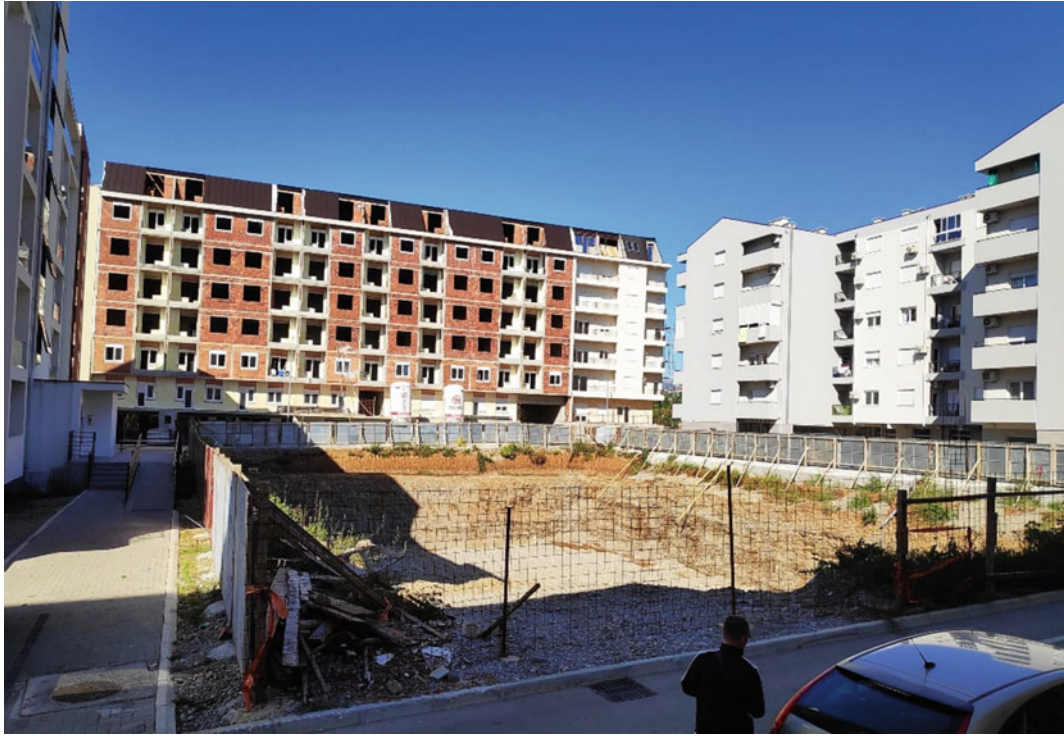
Fig. 18.5 Works on the Ljubović Hill residential building. Source Glas Zabjela (2020)
