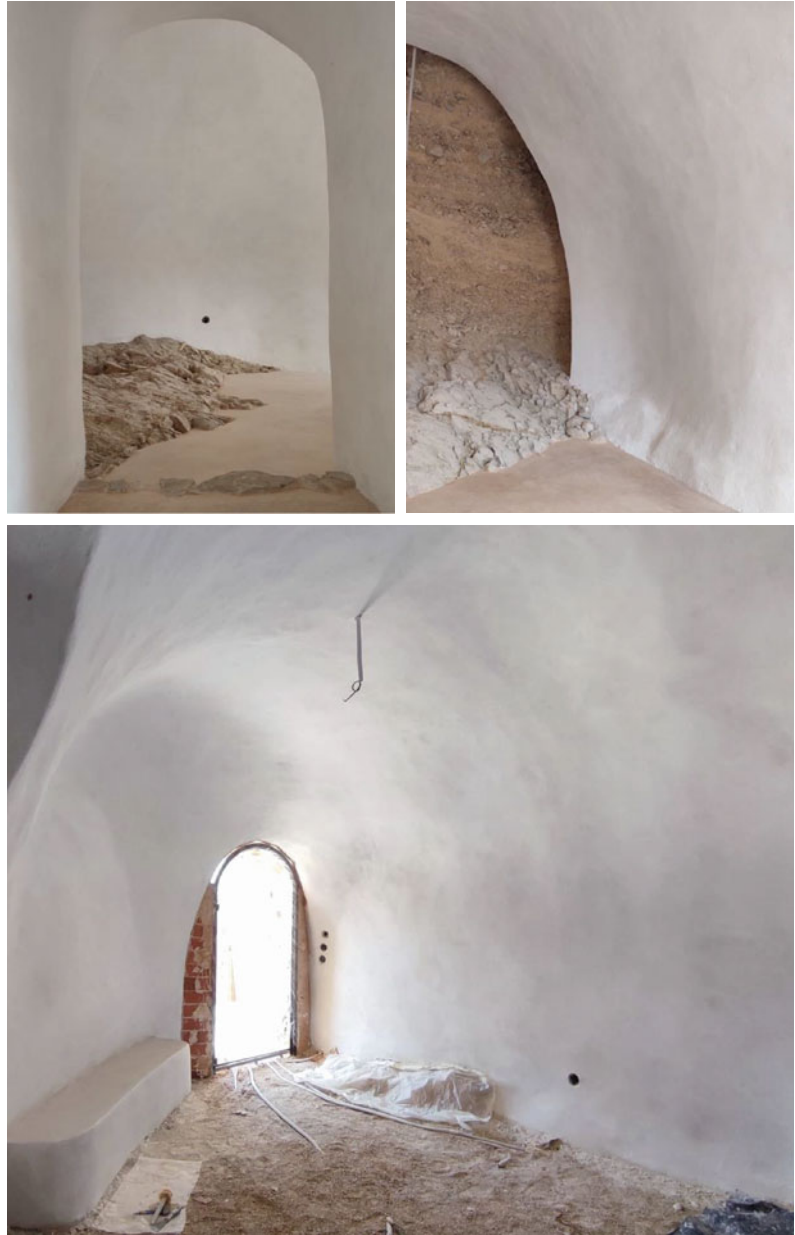
Fig. 19 Vaults after plaster rendering
