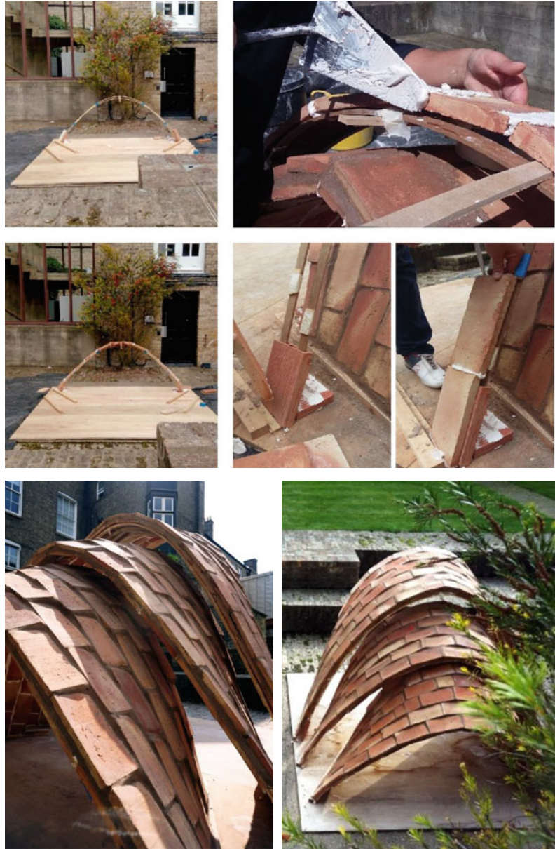
Fig. 10 In situ, vaults prototype by bamboo strips as guidework 2016
