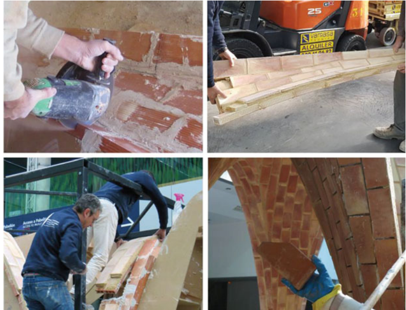
Fig. 5 Construction process of fabricarte
