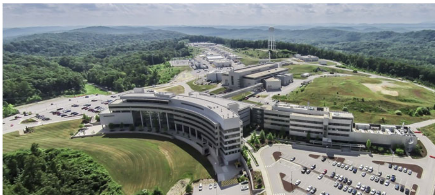
Fig. 1.5 The Spallation Neutron Source. The target building (also known as the experiment hall) is just above center in the photo, and the laboratory and office complex is in the foreground. The linear accelerator can be seen just above the target building, extending approximately 330 m into the background [3]
