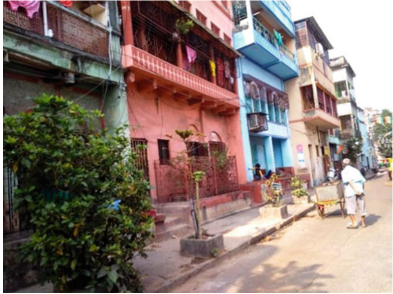
Fig. 11.11 Mid-rise houses in residential neighborhood have higher proximity with street. © Photo Credit: Dr. Shreya Das (Author)
