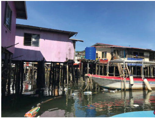
Fig. 4.3 Homes and boat jetties are made of timber materials. Source ACT Malaysia
