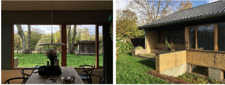
Fig. 14.5 Big trees and the overhanging roof of the detached house from 1973 provide sun shading in summer. The displaced facade creates an enlarged overhang above the bedroom preventing it from overheating
