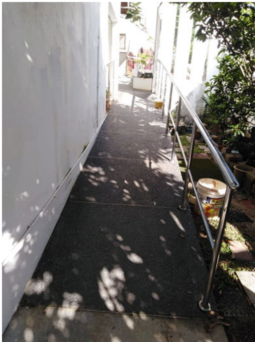
Fig. 20.5 Ramp, crucial element for wheelchair users
