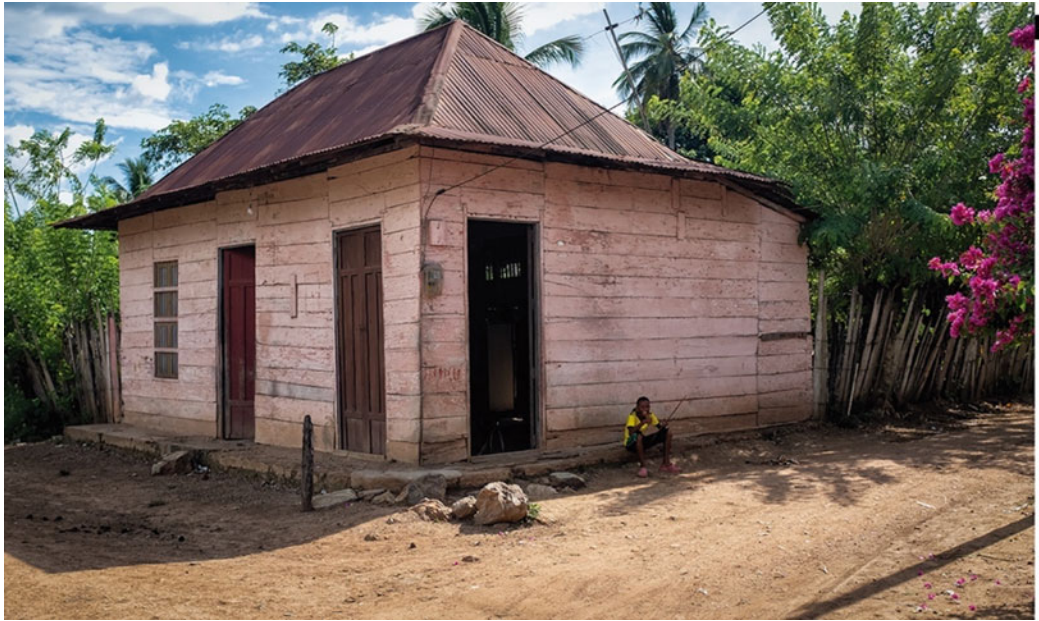
Fig. 6.11 Traditional wood board house. Ma-Majari Community of El Nispero, Montes de Maria, Colombia 2019. @Daniel Huertas
