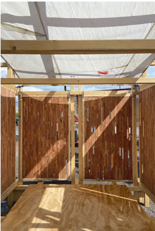
Fig. 12.17 Douglas fir strips are butted to present their expressive end grain. Apertures in the panel arrangement frame views of the landscape beyond. Image ©
