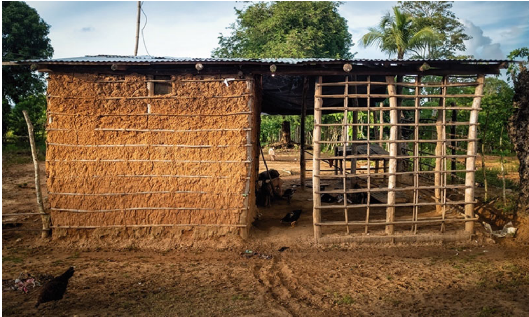
Fig. 6.12 Traditional construction system in “bahareque”. Ma-Majari Community of El Nispero, Montes de Maria, Colombia 2018. @Daniel Huertas
