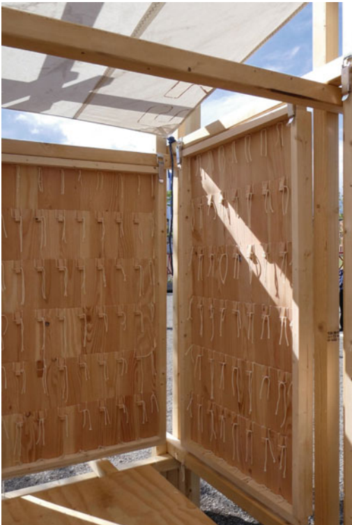
Fig. 12.14 Smell pavilion; interface detail illustrating roof, beam and cladding arrangement. Sensory panel system fixed with proprietary stainless-steel suspension system. Image ©
