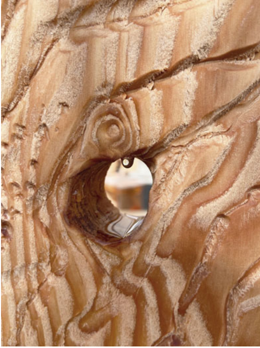
Fig. 12.24 A natural fault in the Douglas timber facade element; machine processing and natural form combined to graphic effect. Image ©
