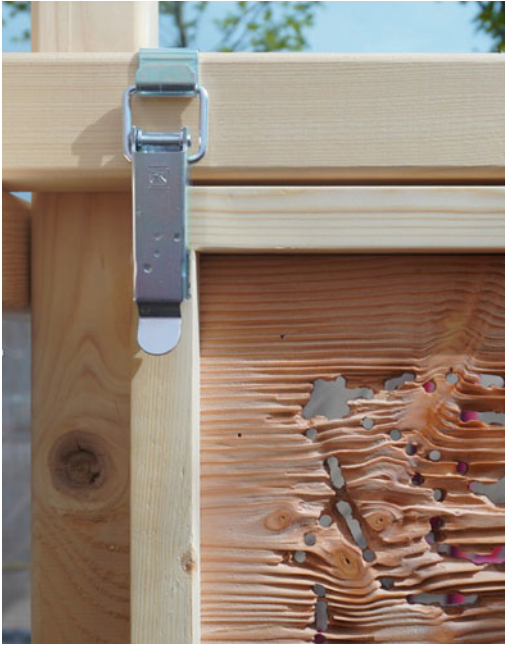
Fig. 12.2 Haptic façade panel displaying natural faults in the wood suspended on bespoke aluminium hanging system. ©
