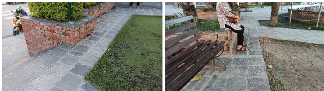
Fig. 18.29 Insufficient width of pathways
