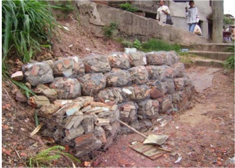
Fig. 42.5 First Mini-Gabion prototype
