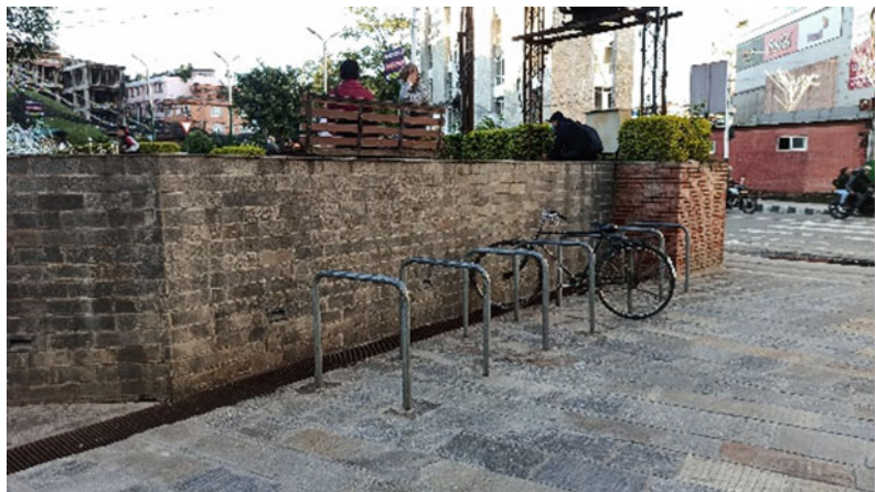
Fig. 18.28 Absence of designated parking spots for PwDs
