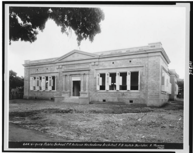
Fig. 7.5 Nechodoma’s public school. Notice the open ventilating windows and shutters to control daylight exposure in the interior/Library of Congress. The image is in the public domain. https://www.loc.gov/item/90710366/
