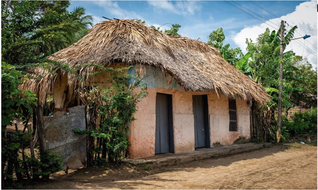
Fig. 6.10 House in “caña parada” (vertical cane), the first house in El Nispero. Ma-Majari Community of El Nispero, Montes de Maria, Colombia 2019. @Daniel Huertas
