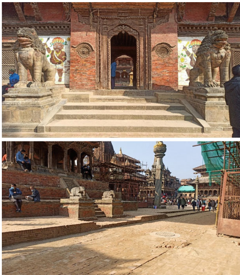
Fig. 18.9 Inaccessible steps without ramps
