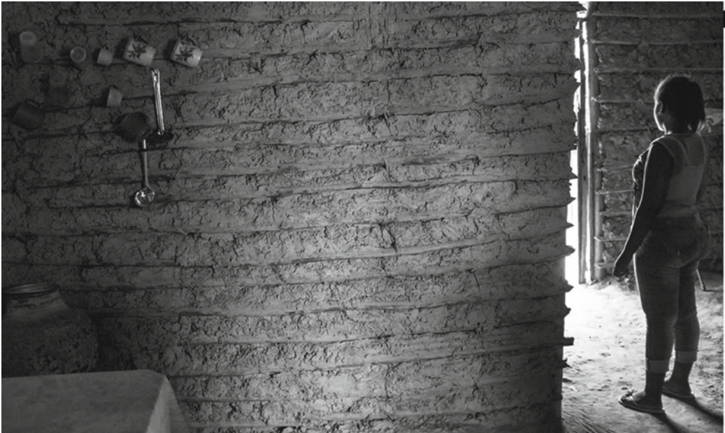
Fig. 6.35 Bahareque interior in an Afro-descendant ancestral dwelling. Ma-Majari Community of El Níspero, Montes de Maria, Colombia 2019. @Daniel Huertas
