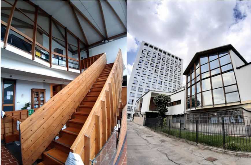
Fig. 2 External and internal views of the Department of Statistics in Florence (Photos G. Manetti)
