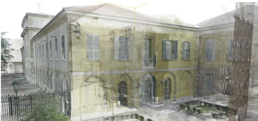
Fig. 5 View of the TLS point cloud within the Cyclone Environment (Editing: A. Dell'Amico, A. Sanseverino, and S. Albertario)
