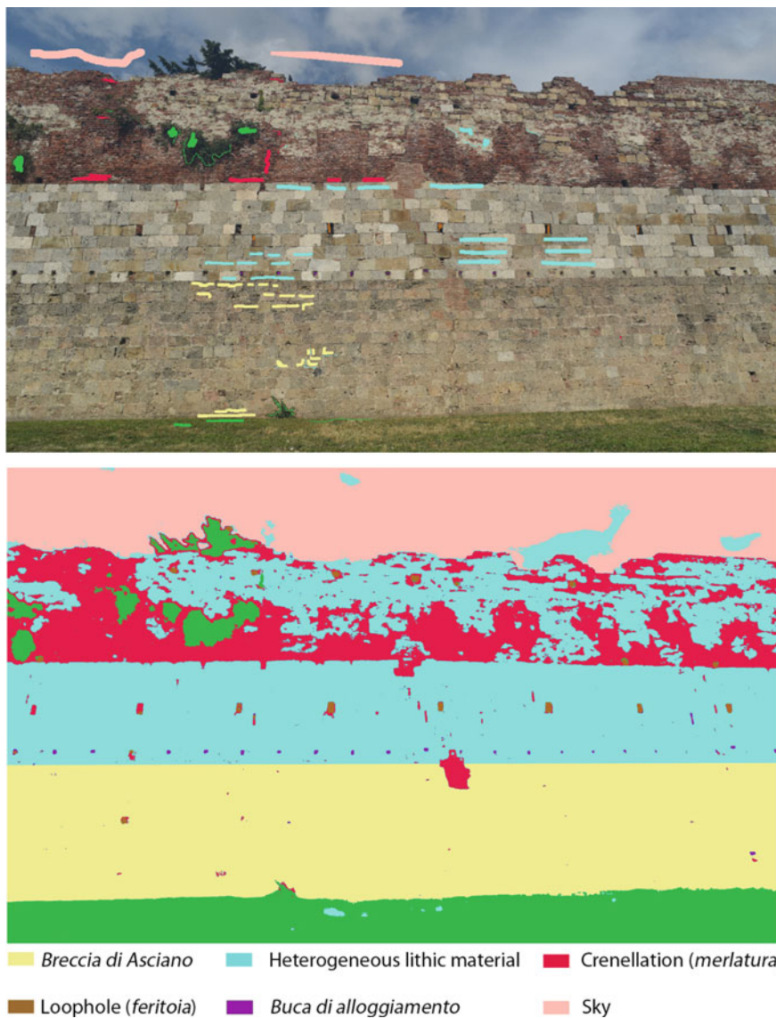
Fig. 4 Manual annotation of a single image (above) and related classification result obtained via the RF (below) for the track in Tersanaia ( Editing V. Croce, M. G. Bevilacqua, G. Caroti and A. Piemonte)
