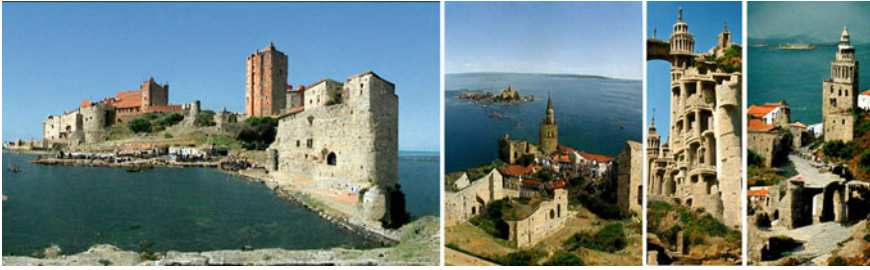
Fig. 16 Same sentence, different frame layout ratios: very different results ( Editing G. Verdiani, P. Arslan and L. Albergoni )
