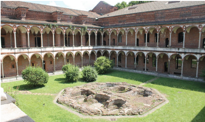
Fig. 2 The Baths courtyard of the Ex Ospedale Maggiore in Milan (Photo F. Banfi, D. Oreni, July 2022)
