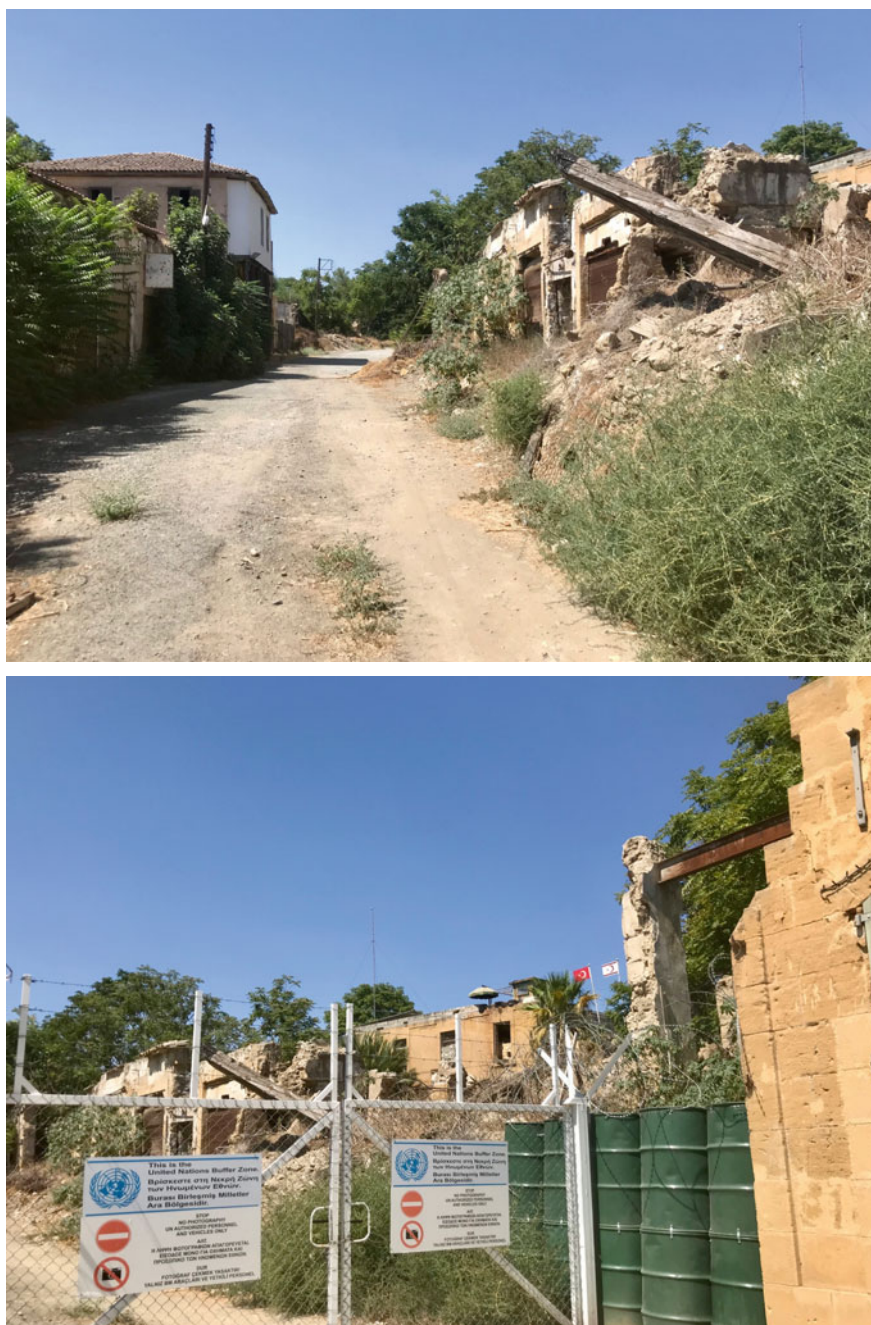
Fig. 3 Built cultural heritage within Nicosia Buffer Zone. Photos by the Authors, 2021
