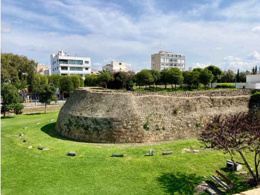
Fig. 3 The Podocataro Bastion and moat. Photo by the authors, 2021
