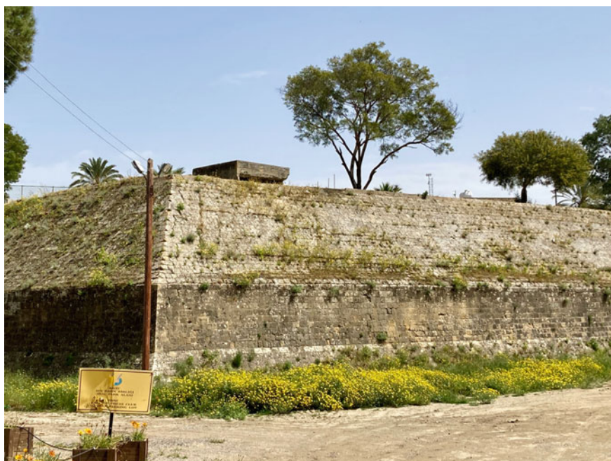
Fig. 4 The Roccas Bastion and moat. Photo by the authors, 2021
