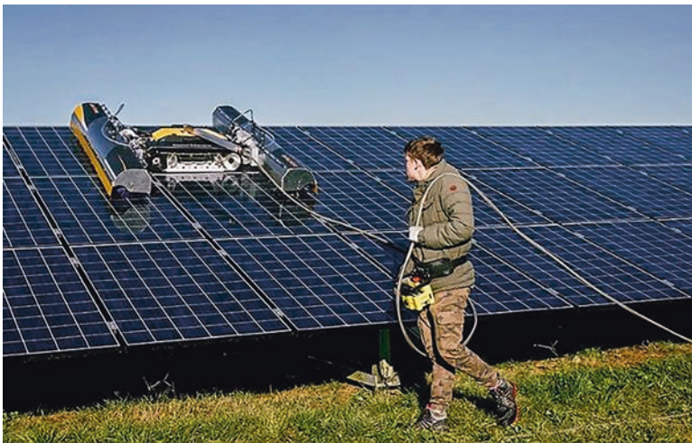
Fig. 11 Maintenance of the photovoltaic modules
