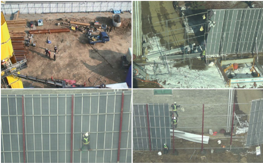
Fig. 4 Construction site scenes of the YUD-COSAv2
