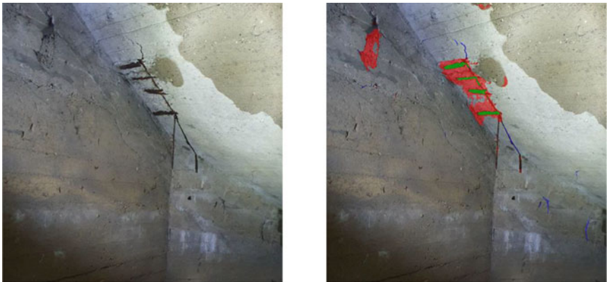
Fig. 8 Segmentation results with the FPN-Effb0 model. Red color masks are spalling predictions, blue color masks are crack predictions, and green color masks are corrosion predictions.
