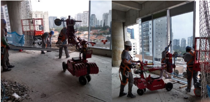
Fig. 10 Transporting and installing frame
