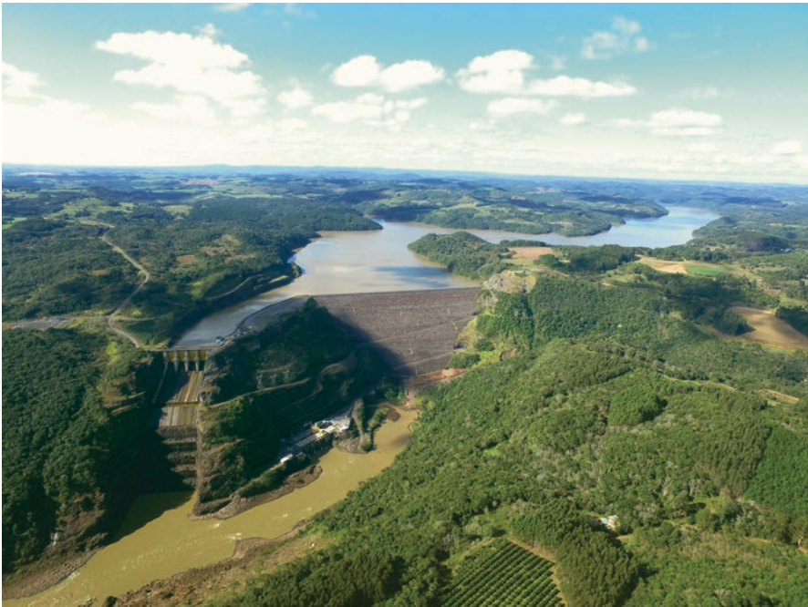
Fig. 12.1 Hydroelectric power plant on the Canoas River, upper Uruguay River Basin, southern Brazil
