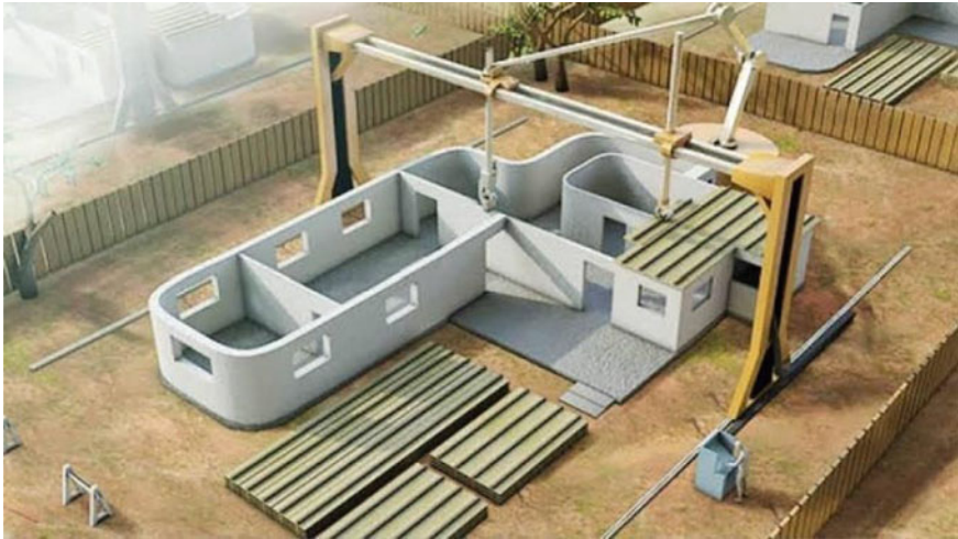
Fig. 1 3D printing in construction
