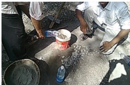
Fig. 2 Mineral water sample was being used to mix the concrete
