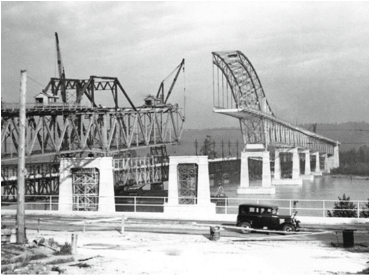
Fig. 8 Construction of Span 2–3, ca. 1937. Source City of Vancouver archives
