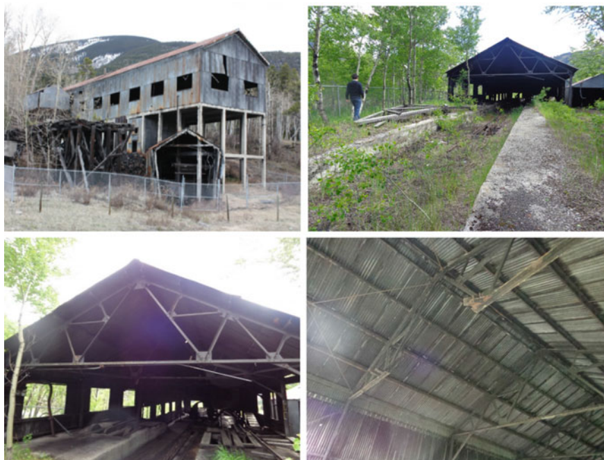
Fig. 3 Views of the Greenhill mine tiple structure from the front and rear above, with a complete roof truss and one missing part of the bottom chord below
