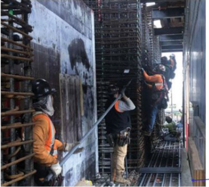
Fig. 2 Crew of five insert #11 (35 M) diagonal bars through wall boundary elements and into a diagonal coupling beam
