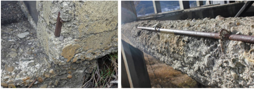
Fig. 8 Reinforcement in a column not spliced to a starter bar in the foundation and shear stirrups in a beam much more widely spaced than one would expect from a modern design
