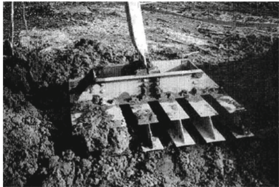
Fig. 1 Full-scale grillage foundation of lattice towers after pullout test [7]
