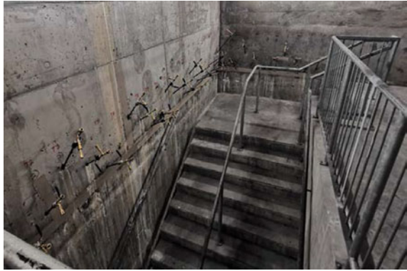
Fig. 2 Injected joint for the in situ tests
