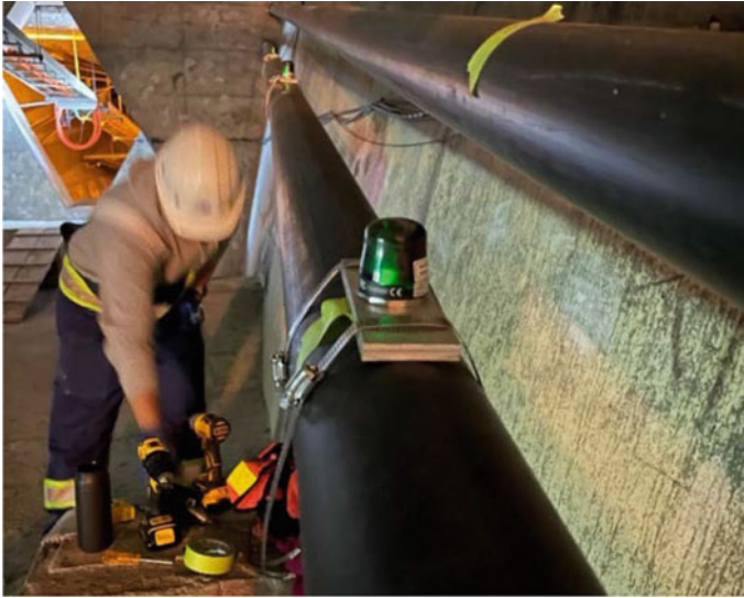
Fig. 3 Sensor installation on tendon
