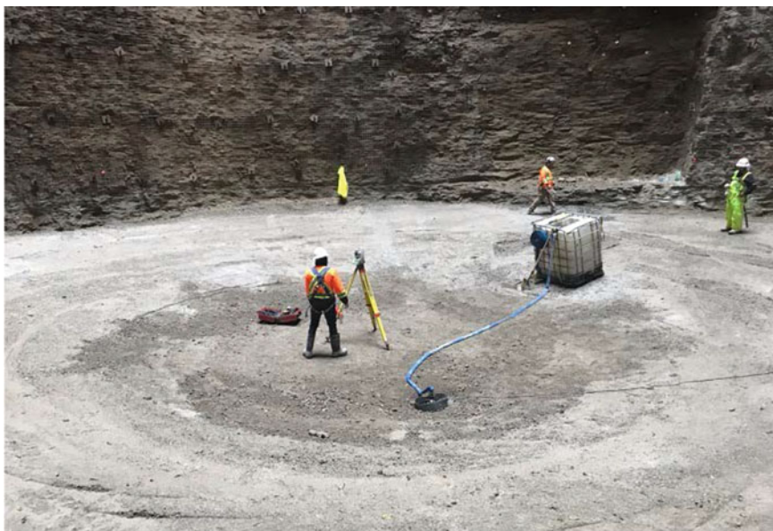
Fig. 4 Hemispherical base slab foundation preparation using accurate surveying and tooling
