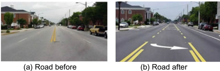
Fig. 3 Road diet on Edgewater Drive in Orlando, Florida. Source Federal Highway Administration
