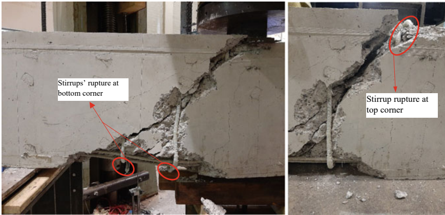
Fig. 15 Failure of beam 2 (shear critical conditioned beam) south face of the beam
