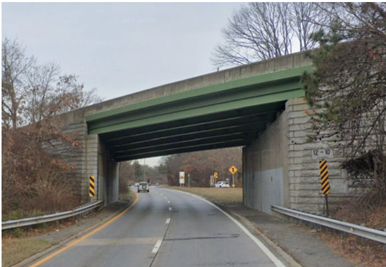
Fig. 3 Photograph of the example bridge (retrieved from https://www.google.ca/maps )
