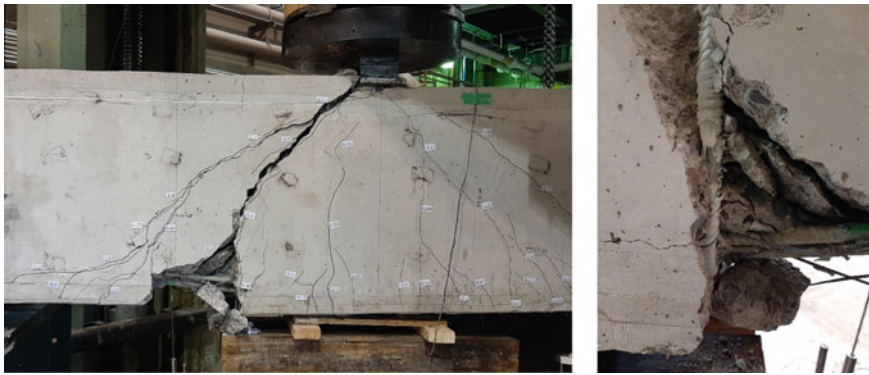
Fig. 10 Control beam failure and stirrup rupture (north face of the beam)
