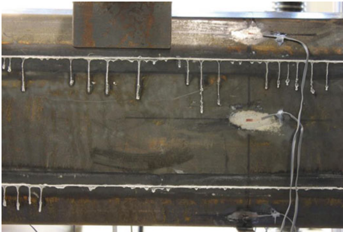
Fig. 6 General view of a fibre optic cable relative to strain gauges
