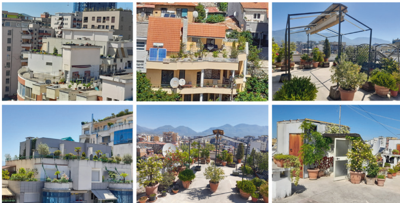
Fig. 6. Existing green roofs in Tirana
