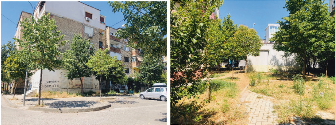
Fig. 7 The potential presence of greenery and the lack of maintenance of a pocket park in Tirana. Source Author
