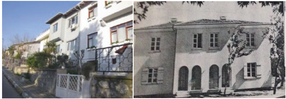
Fig. 6 The bank-houses planned as garden-cities in 1960s, Yapı-Kredi Bank, Kadıköy, Koşuyolu, Asian (Anatolian) and later European, and other districts in Istanbul. Photos, left R. S., 2009 and U. Dogrusöz and IFA Archives
