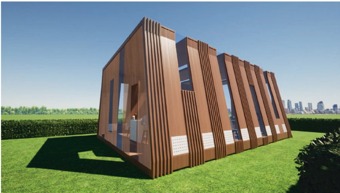
Fig. 16 Final design of the multi-regulation bio-envelope integrated into the pavilion. The figure shows the flat sections of the envelope alternating with the projected ones. It shows the chimney openings on
