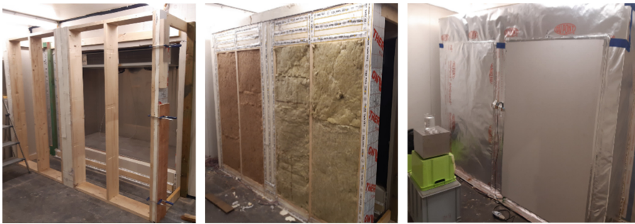
Fig. 4. Walls at different building steps.
