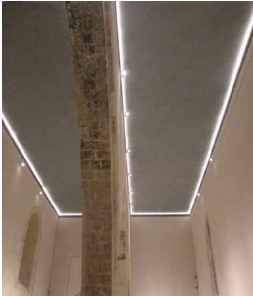
Fig. 17 Weapon room lighting, detail of the lights made by Adragna Illuminazione
