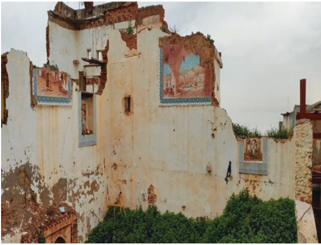
Fig. 7 Picture of a demolished house in the Casbah. Source author 2022
