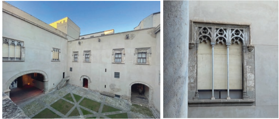
Fig. 1 View of the courtyard of Palazzo Abatellis with the closing of some windows with the fixing of a plywood panel
