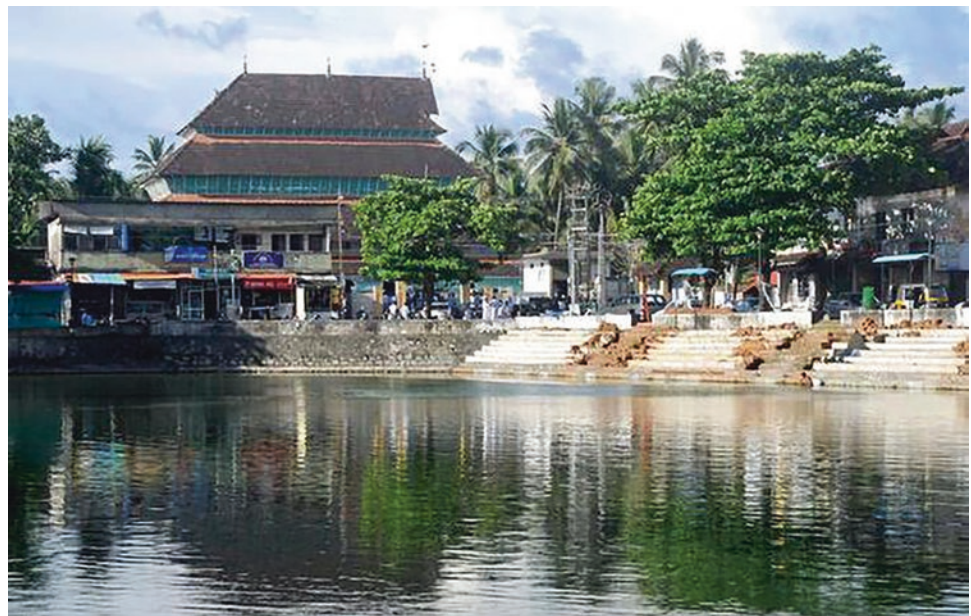
Fig. 9 The historical Kuttichira pond undergoing renovation. (Source K. Ragesh)
