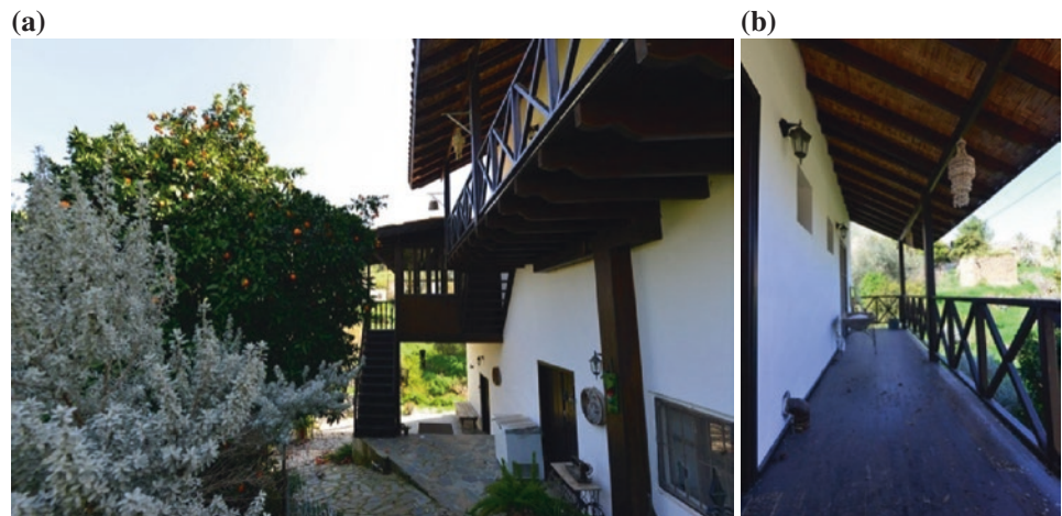
Fig. 6 a Wooden staircase, wooden mid-floor, and wooden balcony b Wooden balcony
