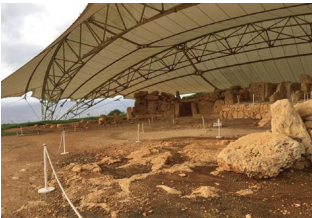
Fig. 11 Malta, Mnajdra, temples protected by a tensile structure, Schillaci (2018)
