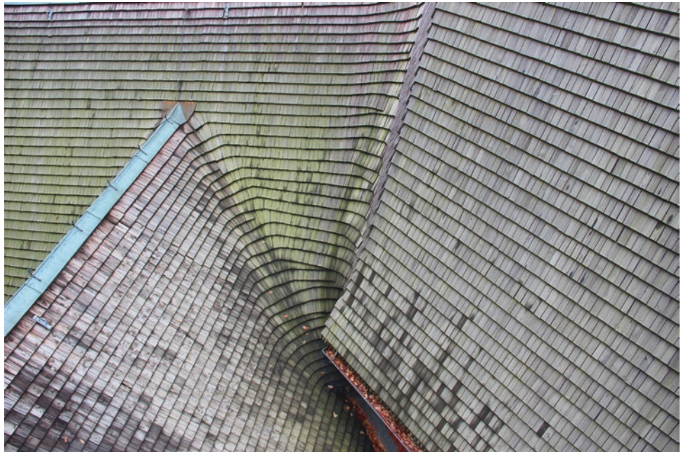
Fig. 8 Curved roof of Kvistbro church. Photo Lisa Skanser
