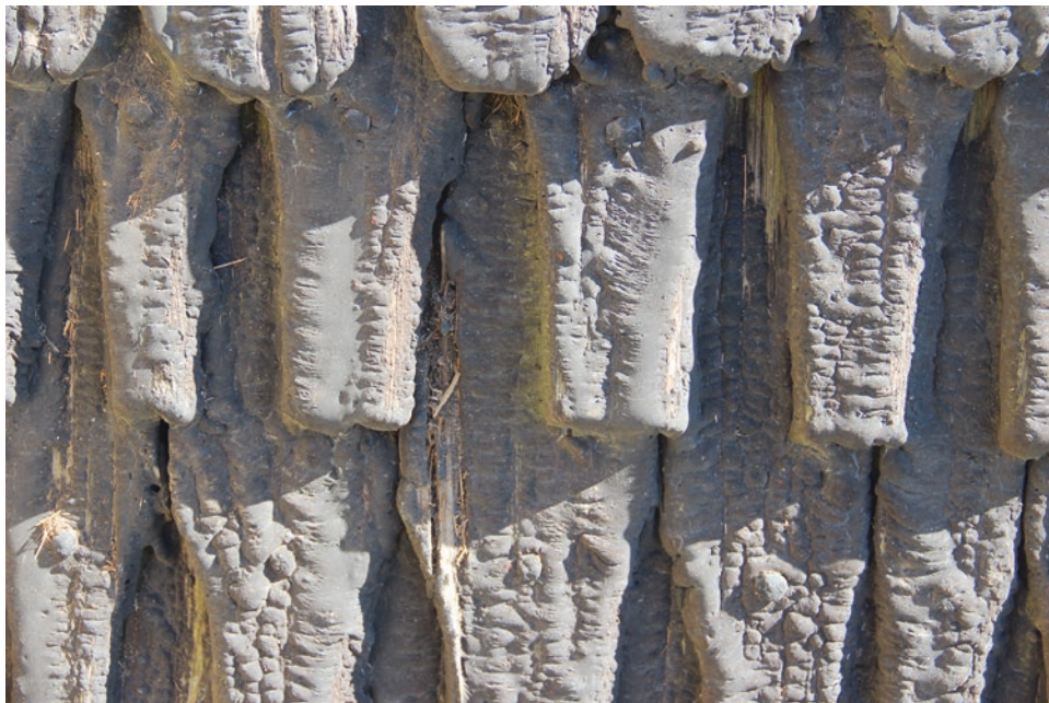
Fig. 7 Thick layer of tar at Sala church. Photo Lisa Skanser
