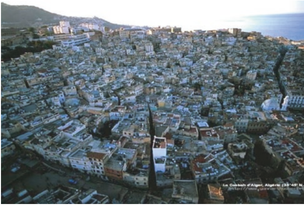
Fig. 3 Integration of the built environment into the morphology of the site. Source National Center for Studies and Applied Research in Town Planning CNERU
