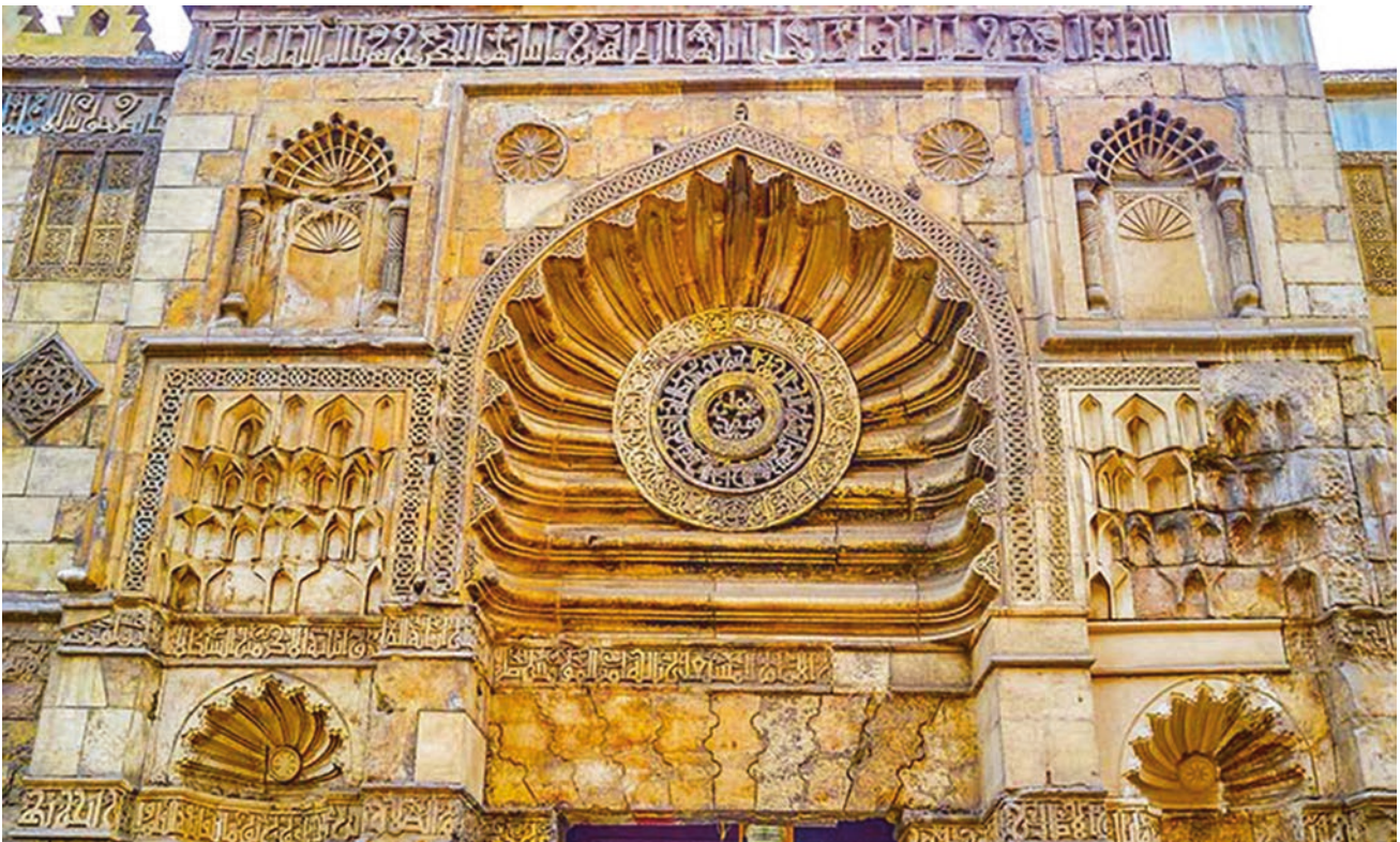
Fig. 1 The main elevation for Al Aqmar showing Muqarnas and oyster
