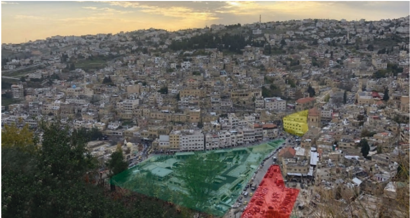
Fig. 11 Oqbe Bin Nafe' project phase 1 highlighted in green, phase 2 highlighted in red and phase 3 highlighted in yellow (ElFaouri, 2020–2021)
