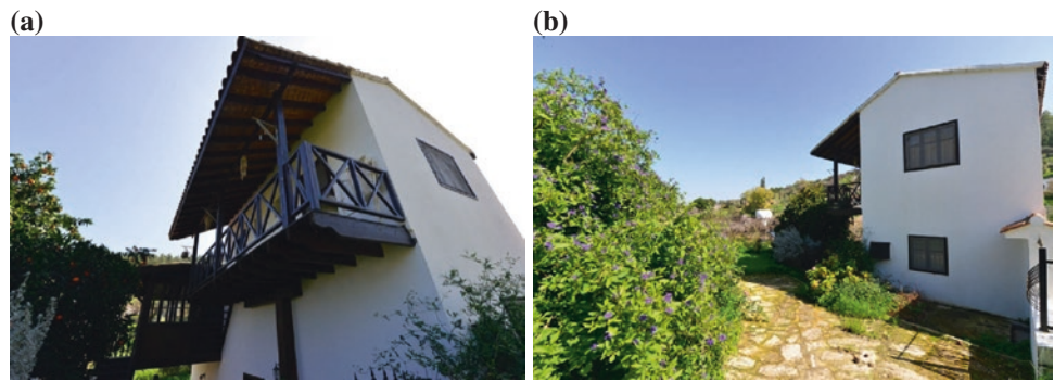
Fig. 4 a Wooden mid-floor and upper floor b Upper floor
