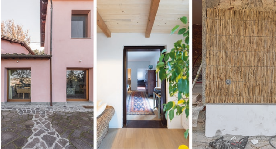
Fig. 2 Building views from left to right: outdoor view, indoor view, detail of reed panels insulation (© Matteo Pierattini)
