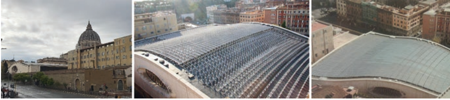
Fig. 4 BIPV roof of the Nervi Hall. (Source: Elena Lucchi and [6])
