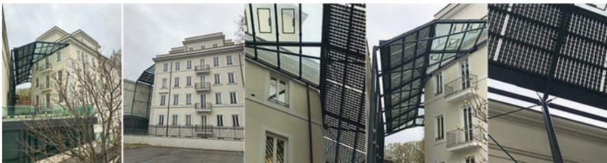
Fig. 6 Glazed PV roof with iron structure of the atrium. (Source: Elena Lucchi)
