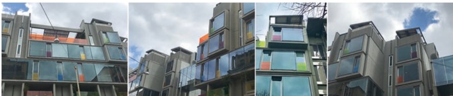
Fig. 5 Façade and PV canopies on the building roof. (Source: Elena Lucchi)
