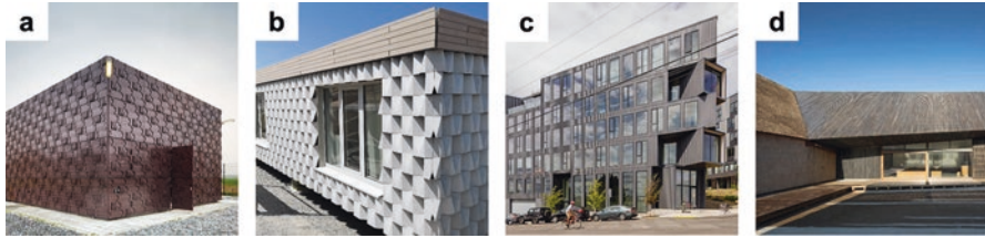
Fig. 5 Existing building where biowaste-based products were used: (a) gas station in Dinteloord (the Netherlands) that is covered by biobased panels based on bioresin and hemp fiber, (b) facades made with panels of road grass, recycled toilet paper and fabrics, (c) Flatiron PDX in Portland (USA) whose façade and floor are made with laminated wood panels. (d) Danish Wadden Sea Center in Okholmvej (Denmark) whose façade and roof were clad using local straw
