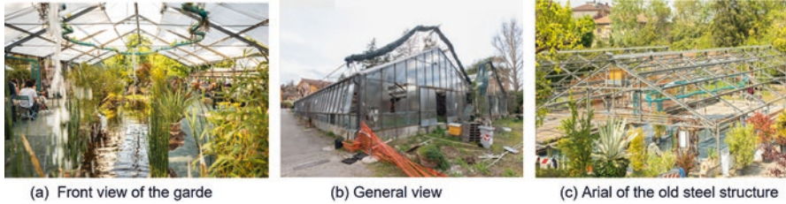
Fig. 2 Existing situation of Le Serre of Giardini Margherita in Bologna, Italy. (a) Front view of the garden. (b) General view. (c) Aerial of the old steel structure. (Image source: developed by authors)
