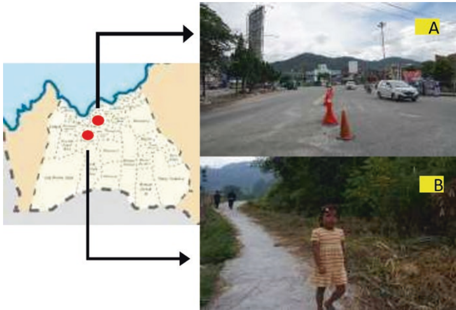
Fig. 8 Street in Balige. (a) Sisingamangaraja Street, Balige. (b) Road in the village of Sianipar Sihail-hail. (Source: Daritoba Project (April 2019))
