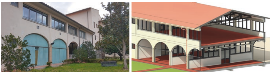
Fig. 1 South façade of the pilot building under renovation in the School of Architecture – Santa Verdiana, Florence and the digital BIM model
