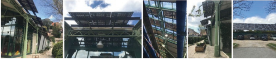
Fig. 2 BIPV brise-soleils and PV car shelter of the Explora Museum. (Source: Elena Lucchi)
