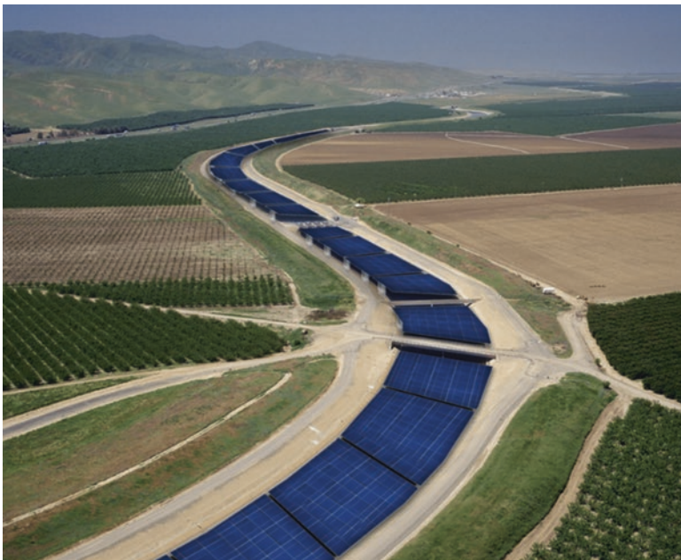
Fig. 12 Solar power canopies over California 4000 m canals could show a savings of 63 billion gallons of water annually, while 13 GW of solar panels could be installed and ready by 2024 [10]
