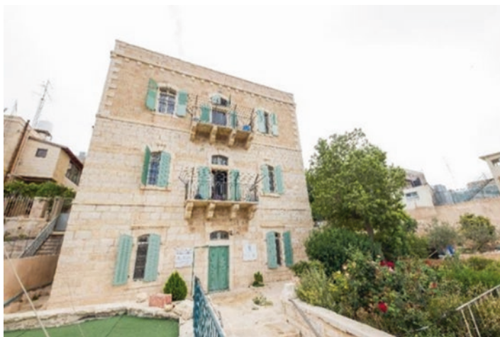
Fig. 1 Case study building
