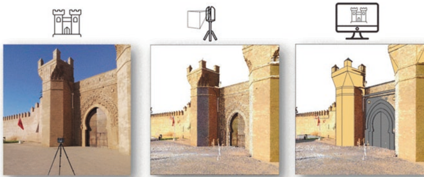
Fig. 4 Scan-to-BIM: From left to right: Left: The survey of Chellah’s gate using a Faro Laser scanner. Middle: The resulting point cloud. Right: The BIM model overlaid on the point cloud
