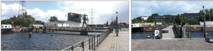
Fig. 3. Views of Citadel Bridge, Hamburg, Germany
