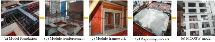
Fig. 6. Construction process of the MCOSW model.
