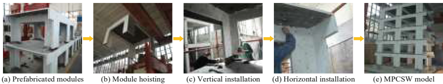
Fig. 5. Construction process of the MPCSW model.
