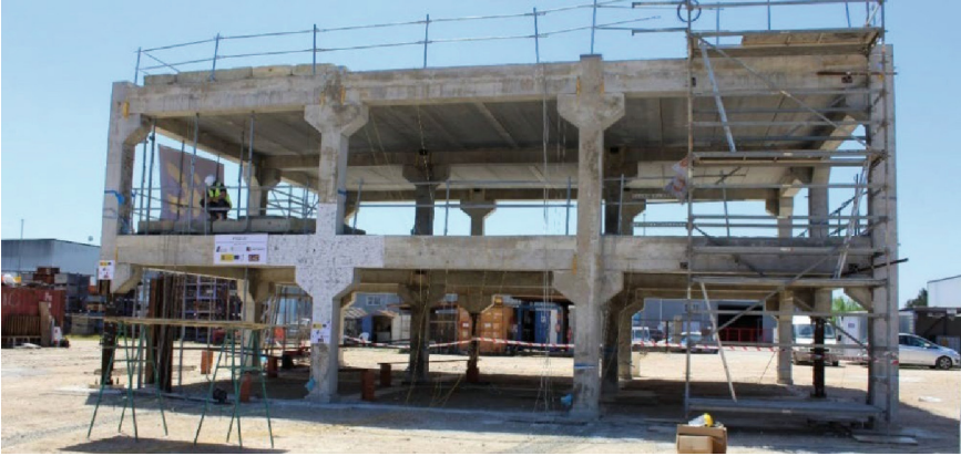
Fig. 3. Completed building specimen prior to testing.
