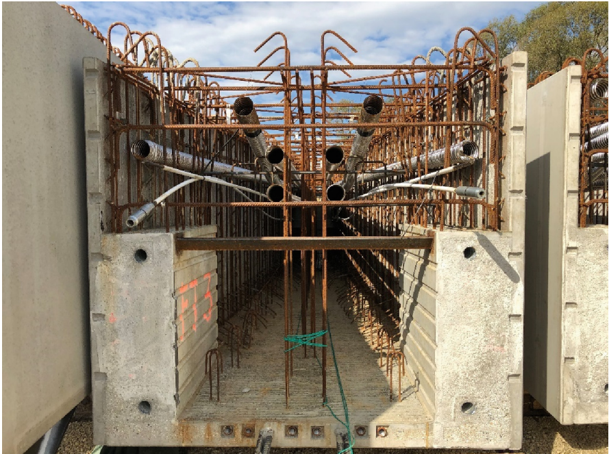
Fig. 1. U-shaped thin precast element for a bridge girder
