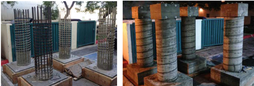
Fig. 2. Rebar cages and finished columns.
