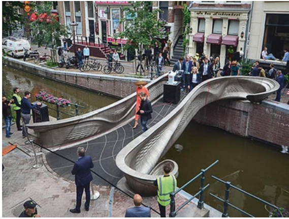
Fig. 8.3 MX3D Bridge. (Photo by Adriaan de Groot)
