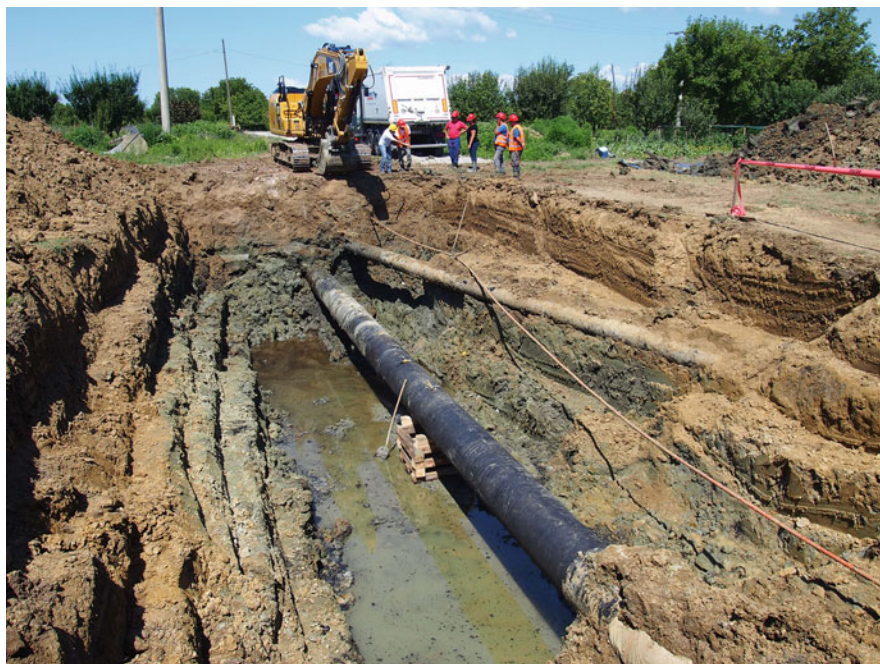
Fig. 15 Example of anthropogenically induced soil contamination. Ruptured gas and oil pipeline as a source of soil contamination near Garčin (Photo taken by Ivica Kisic, July 2019)
