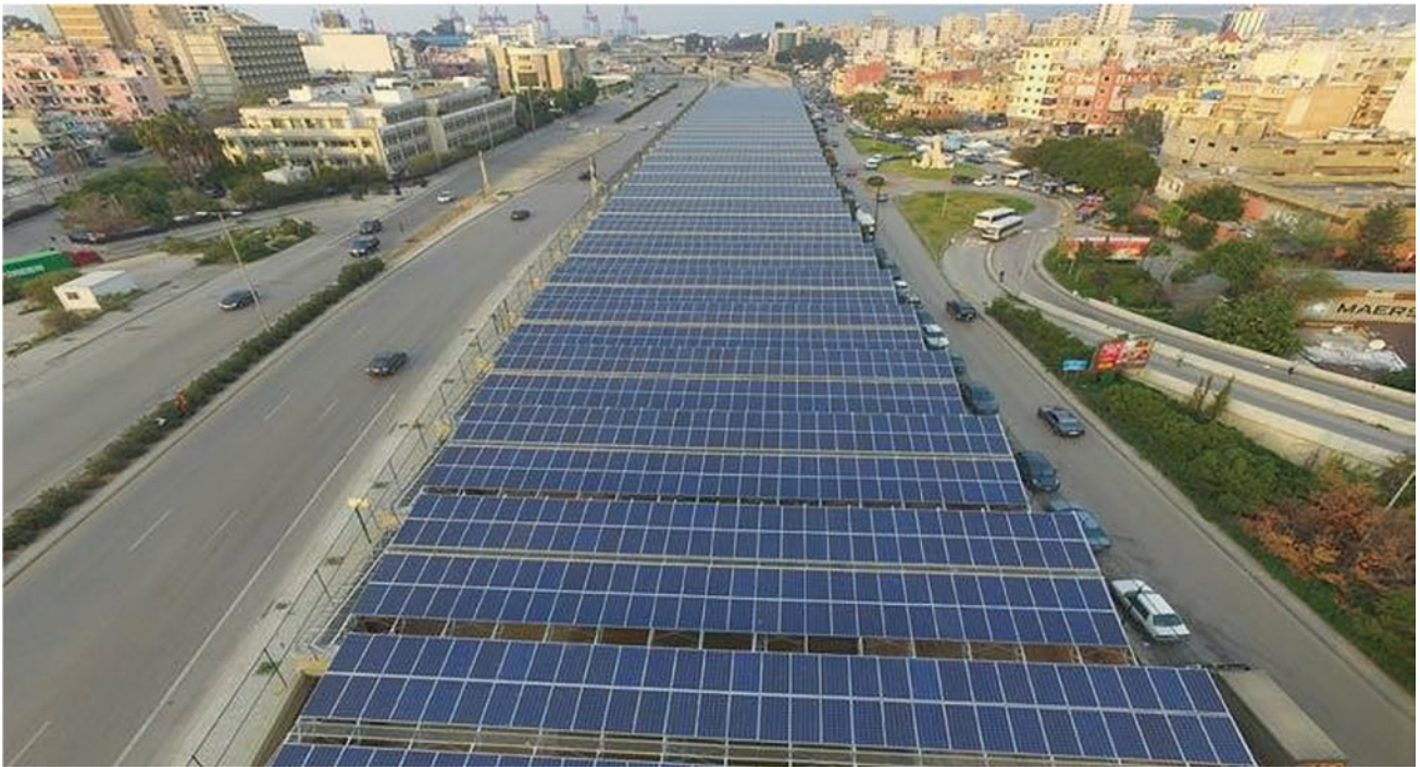
Fig. 5 Beirut River Solar Snake PV installation [3]
