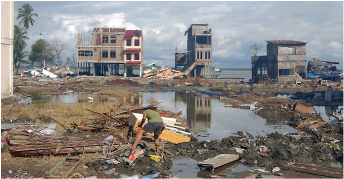
Fig. 6 Aftermath of 2004 earthquake tsunami in Meulaboh, Indonesia. (Photo by Jennifer Rivera. Public domain [56])
