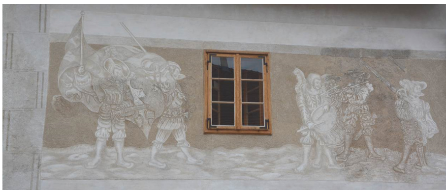
Fig. 8. The reconstructed sgraffito facade after two years. Slavonice, house No. 545.
