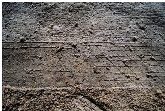
Fig. 2. Detail showing three basic surface finishing techniques of the sgraffito. In the upper third, the lime wash is untreated and this finish acts as the brightest one, in the middle third, the lime wash is partially removed and smoothed with a spatula. This surface was subsequently decorated with hatching. The darkest part at the bottom was created by completely scraping away the lime wash and partially also the mortar surface.
