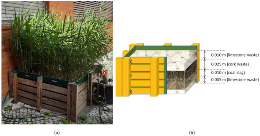
Fig. 15.1 Picture of the CW prototype (a), and schema showing the filling media consisting in four layers of three recovered solid wastes (b)
