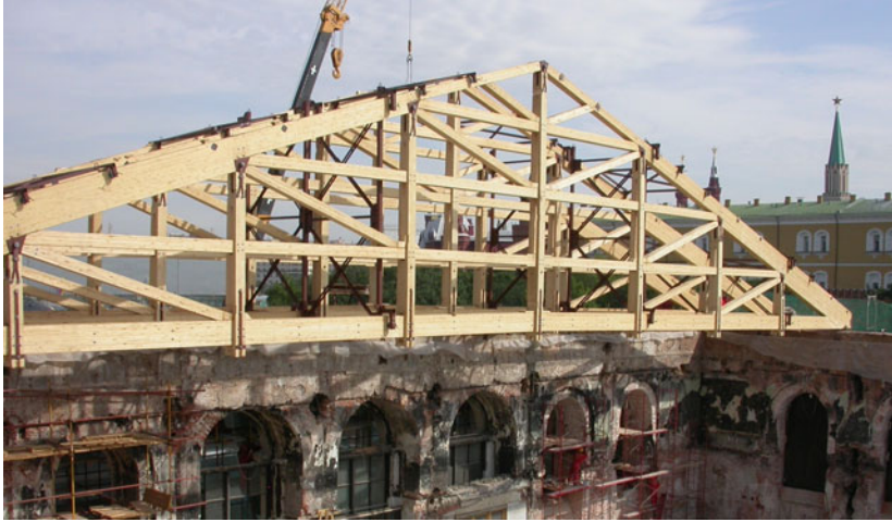
Fig. 5 Assembly of the Manezh Central Exhibition Hall trusses
