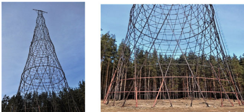
Fig. 1 A unique hyperboloid support for the 110 kV overhead line crossing over the river. Oka 128 m high, erected in 1927–29 on the left bank 12 km from Dzerzhinsk, Nizhny Novgorod region (photo by the author, 2014)
