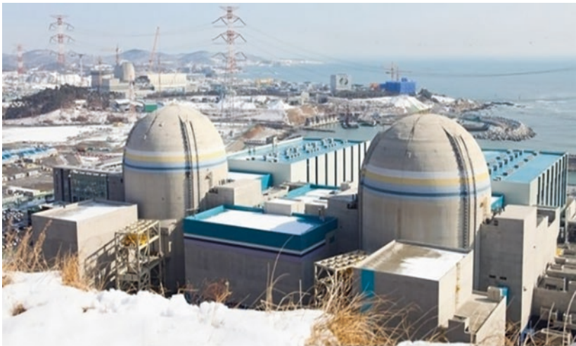
Fig. 1 Example of a nuclear power plant: Kori Nuclear in Korea
