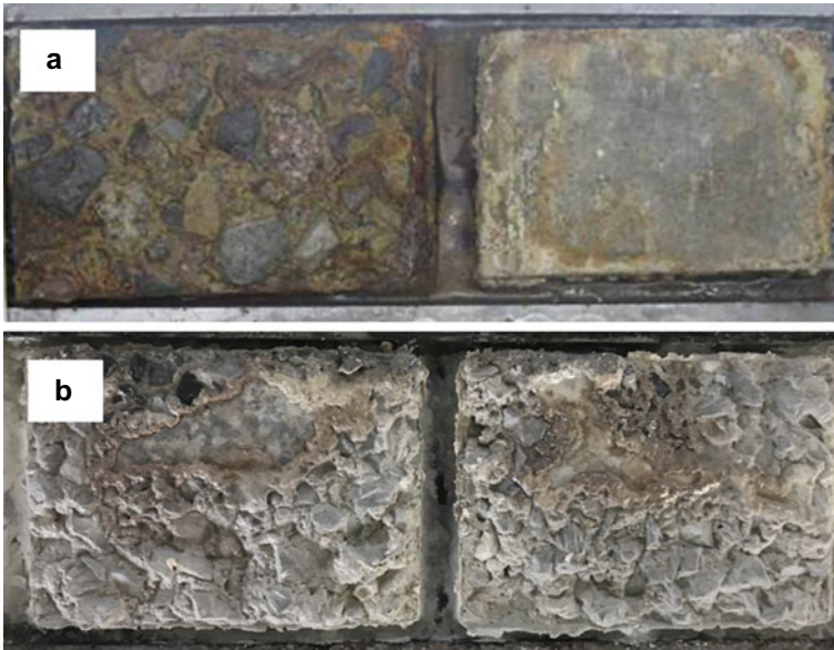
Fig. 5 Surface characteristics of two OPC concrete (a) and calcium nitrite admixed concrete (b) samples after surface washing
