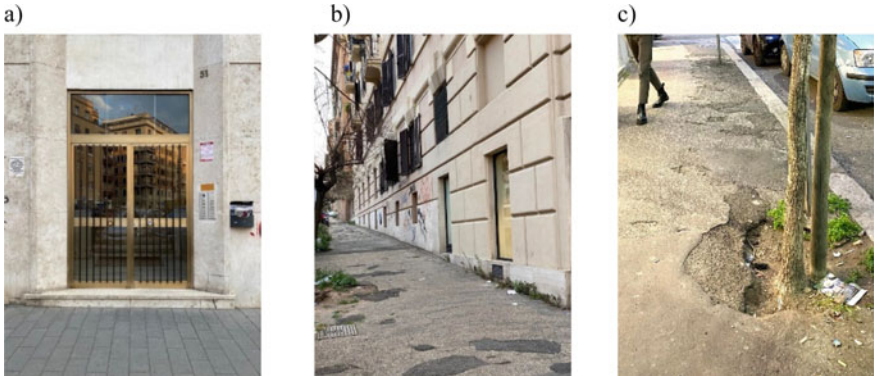
Fig. 85.2 Walkways in the case study. a An architectural barrier at building entrance in Via Urbino. b Irregular surfaces in Via Fregene. c Incompliant gaps in Via Veio
