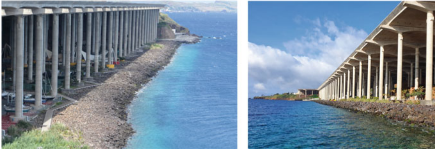
Fig. 1 General view of the berm breakwater and the foundation columns of the airport runway extension, April 2021
