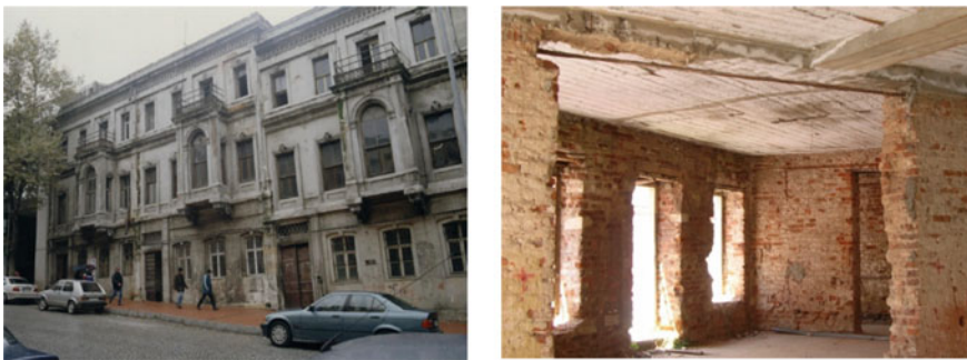
Fig. 1 Akaretler row houses, load-bearing masonry walls and RC floors [8]
