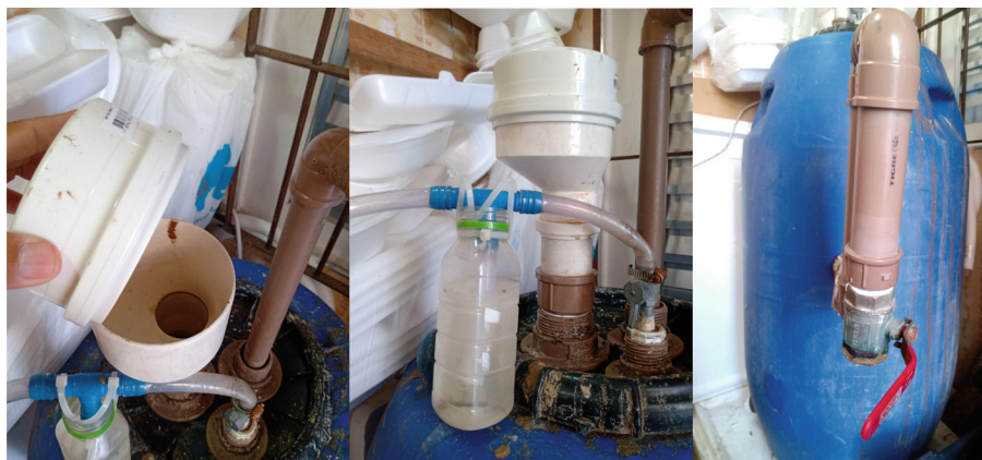
Fig. 3. A) Improvements of the reactor feed inlet B) and safety valve C) improvement in the exit of the digestate
