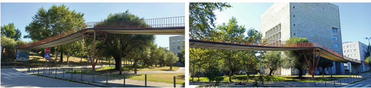
Fig. 1. Views of the FEUP stress-ribbon footbridge.
