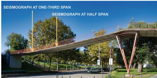
Fig. 3. Location of the two seismographs used for the data collection process, positioned at one-third and a half of the longest span of the footbridge.
