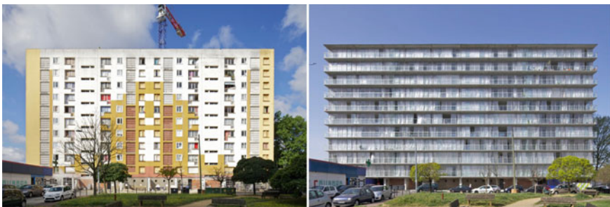
Fig. 12.3 Transformation of 530 dwellings, Bordeaux. Courtesy of Philippe Ruault
